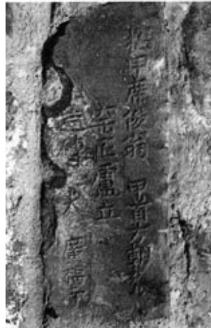
2.3 Lu Li's brick is currently embedded in a Nanjing city gate. The inscription on the brick reads:
