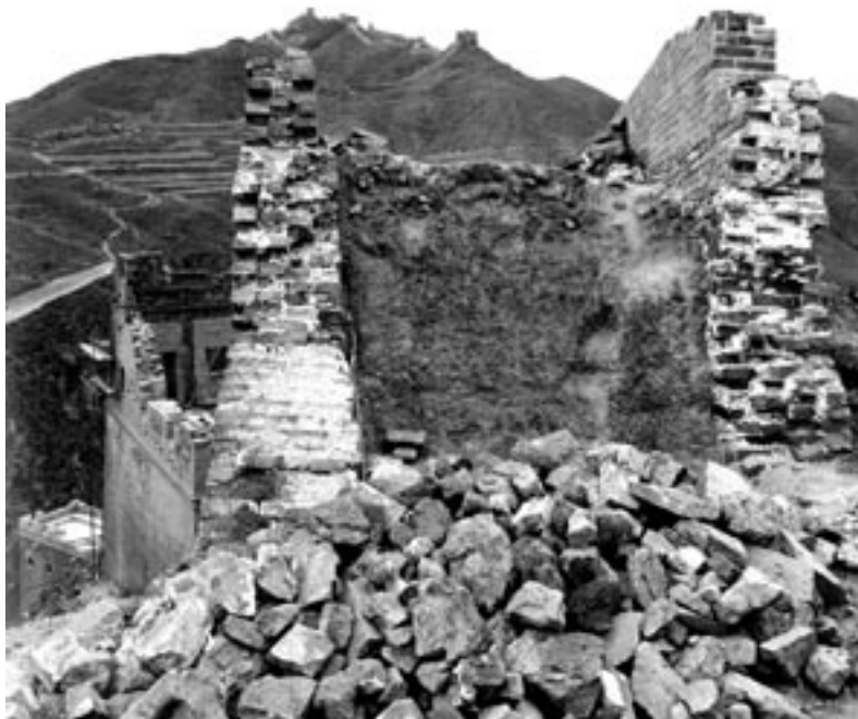
3.17 The cross section shows the solid mud core of the Wall.
