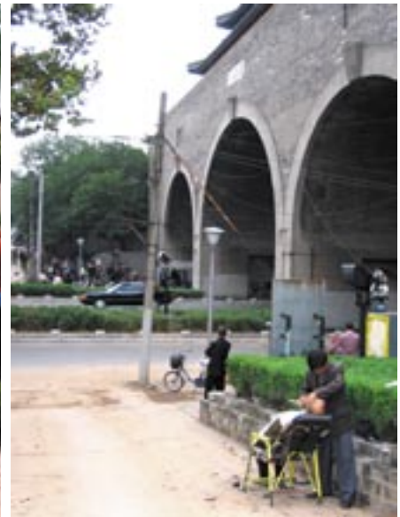
A13 Street barbering at the foot of the gate. The day I visited this Yijiangmen, there were also local people gathered at the foot of the gate playing card games. [10.21.2005]
