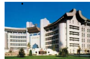
Capital Library completed in 1999
