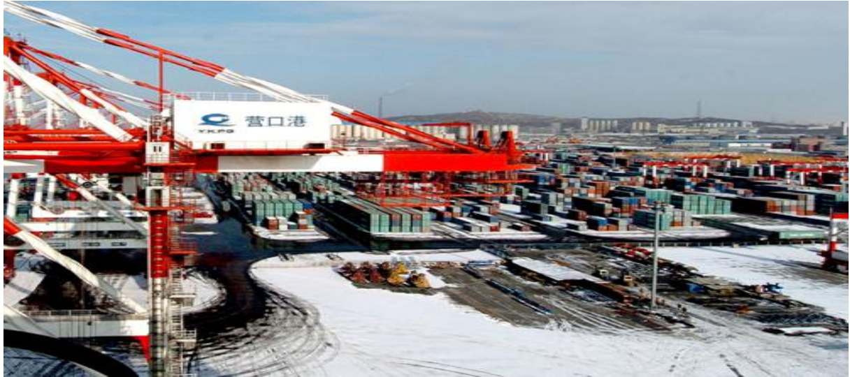
Figure6-7: Current Situation of the Port of Yingkou (2005)
