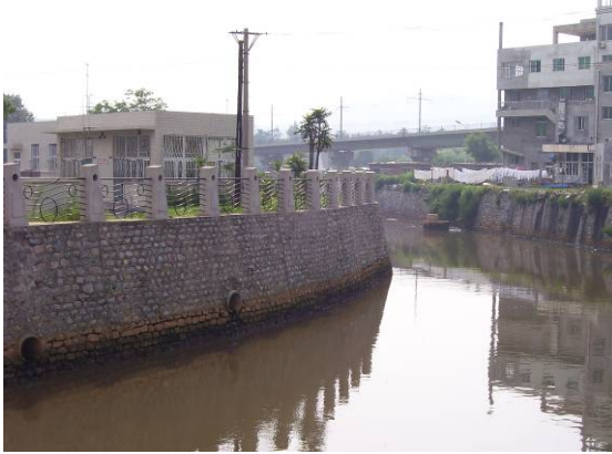
Lingshui River and nearby Sewer Pipes
