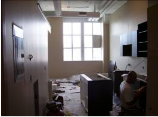
Loft being furnished
