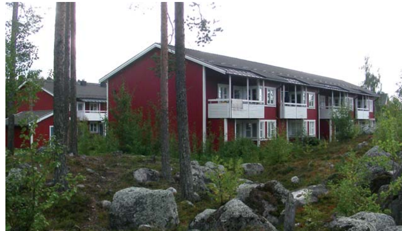
Fig. 4.7 Townhouses in Storuman, Sweden. The red paint is noticeable as a regional aesthetic; traditionally the red colour emerged from an iron oxide paint mixture, which was used to protect the exterior wood cladding. The iron oxide was a waste by-product of iron ore smelting plants.
