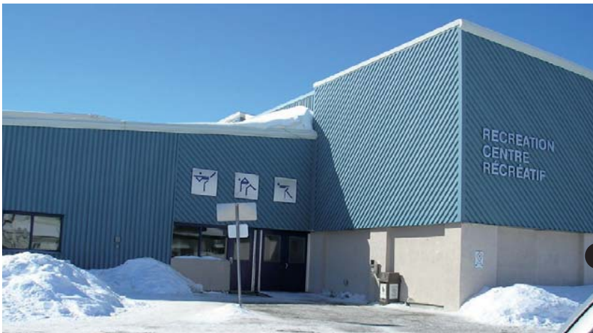
Fig. 5.4 Photographs 5-7, the public high school and elementary school and the recreation centre respectively, are key institutions for community youth. In Chapleau, the built environment does not effectively engage the youth with respect to local forest resources or innovative places. The bottom two images depict the interior of the recreation centre: left, the lounge adjacent the curling rink and right, the projection screen used to show community movies.
