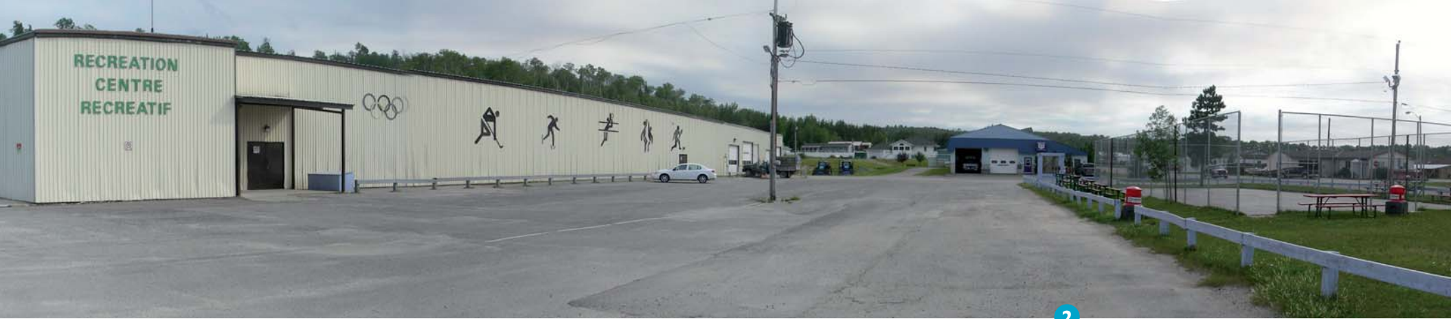
Fig. 2.6 Photo documentation and housing statistics, Dubreuilville. Views located on aerial (Fig. 2.5).
