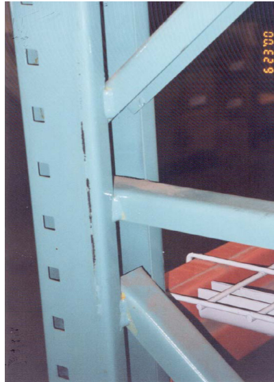
Figure 6-6: Typical rack bracing members and connection (NEHRP, 2003)
