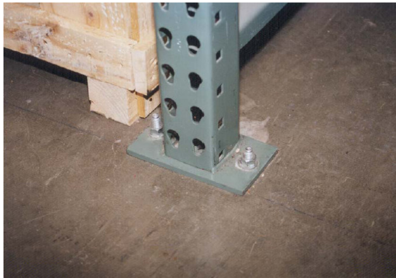
Figure 6-7: Typical column base plate connection (NEHRP, 2003)
