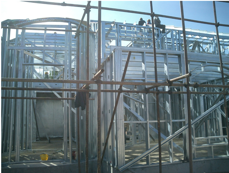
Figure 2-3: Cold-formed steel framing—Example 2
