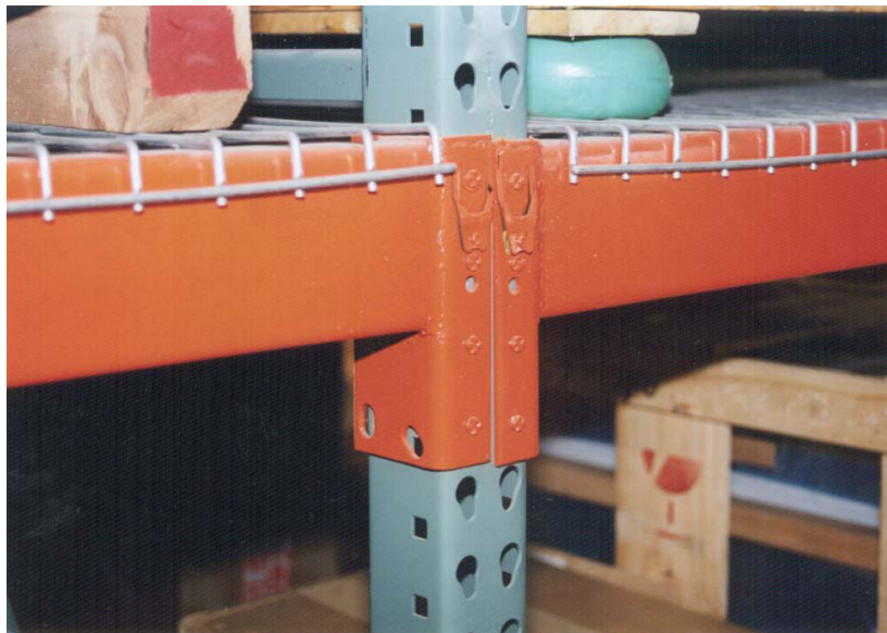
Figure 6-5: Typical rack moment connection (NEHRP, 2003)
