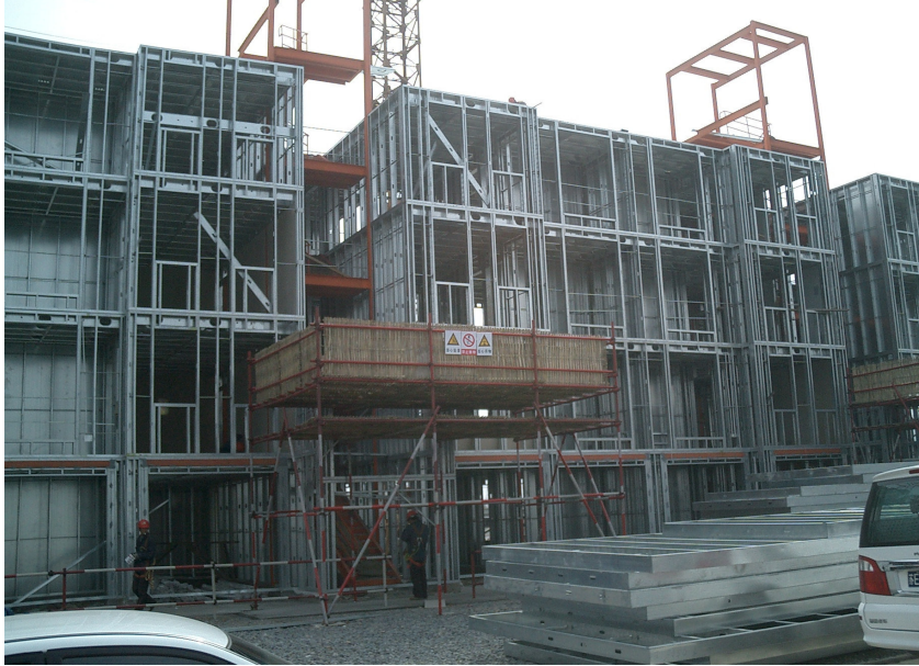
Figure 2-2: Cold-formed steel framing—Example 1
