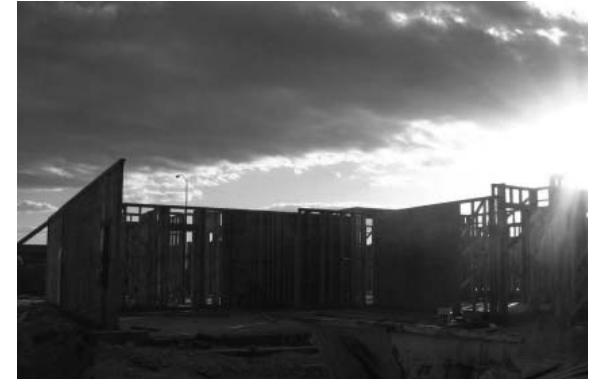
Fig. 1.3 - Home is more than this.
