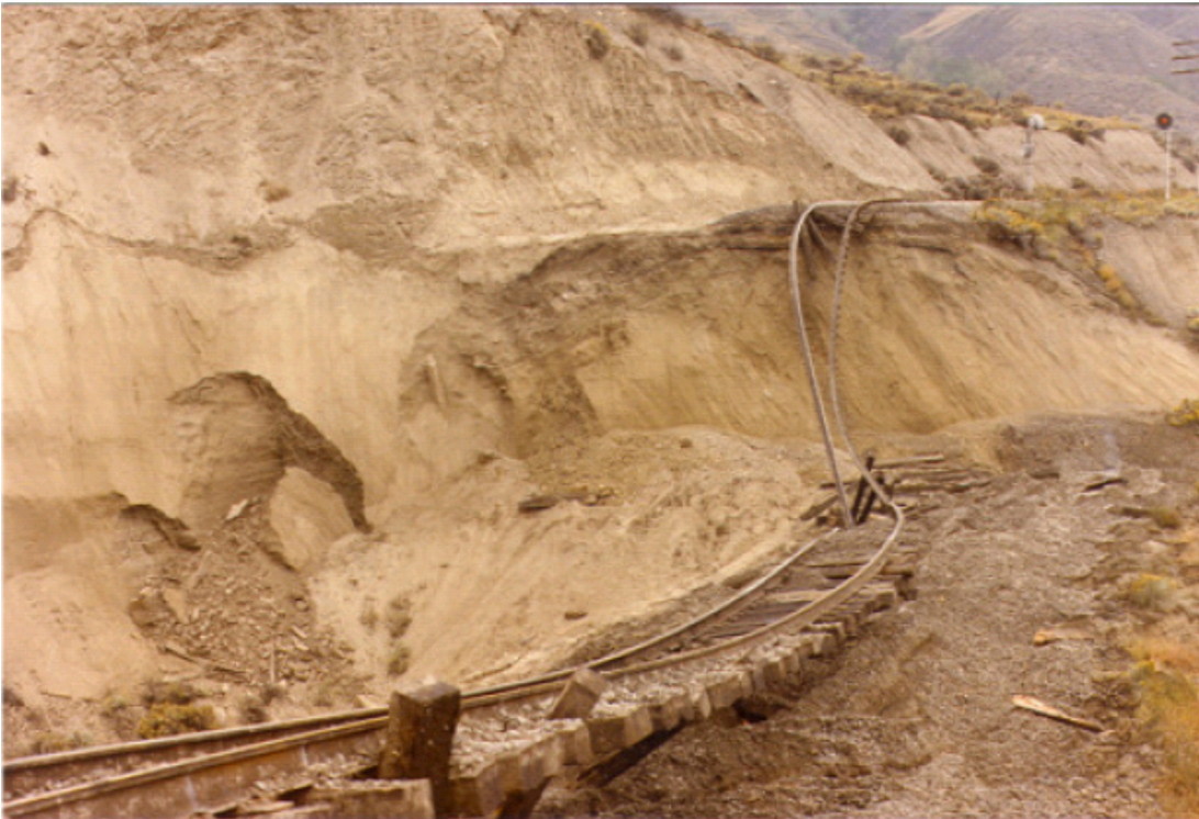
Figure 1 - 3. Photograph showing destruction of CP rail lines caused by the movement of the 1982 Goddard landslide. Top: deformation in the rail along the eastern edge of the landslide. Bottom: severance of the rail line caused by differential landslide movement. Photos used with permission from Chris Bunce, CP.
