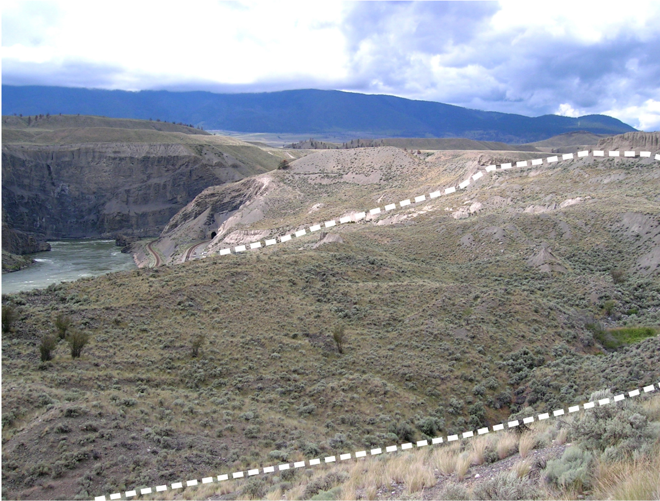
Figure 1 - 4. Photograph looking northwest above the present-day South Slide. Dashed lines show the approximate extent of the landslide debris. Movement is towards the river (to the left).
