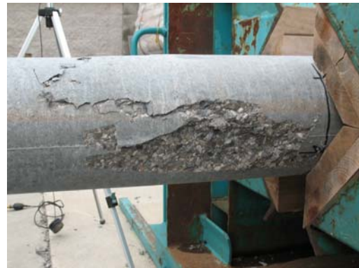
d) Crack pattern (loading side)
