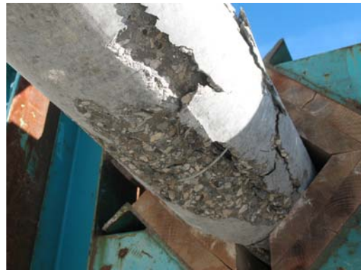
d) Failed section at butt (from bottom)
