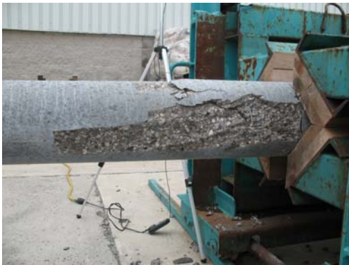
c) Failed section at butt (loading side)
