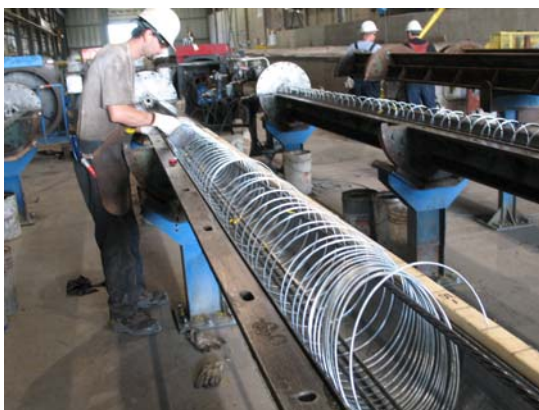
Figure 4.14: Placing the helical reinforcing
