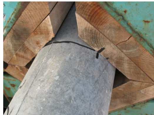
d) monitoring movement at pole clamp end
