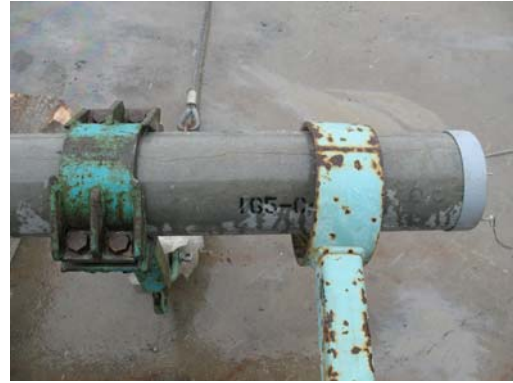
b) Longitudinal cracking along strand
