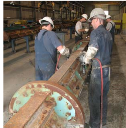
Figure 4.17: Tightening bolts on mould
