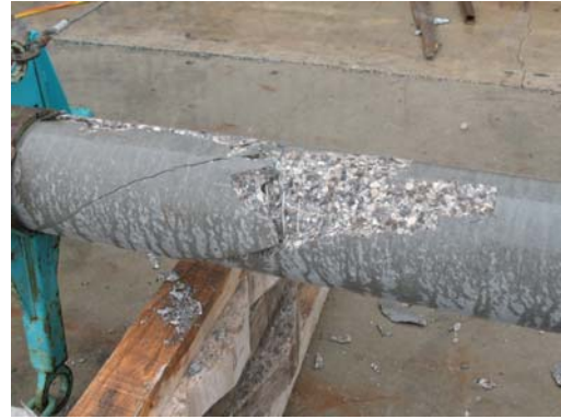
b) Loading collar failure (loading side)
