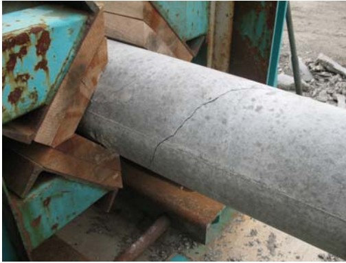
a) Initial cracking at butt
