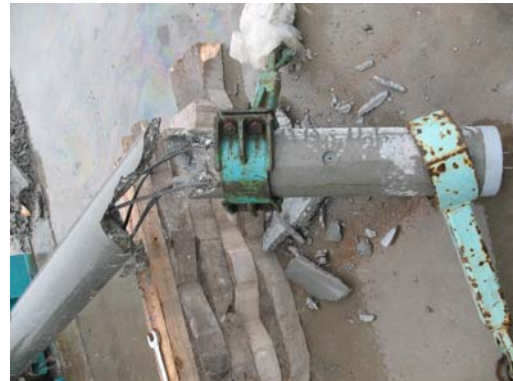
f) Ultimate failure of 165-C-2 specimen
