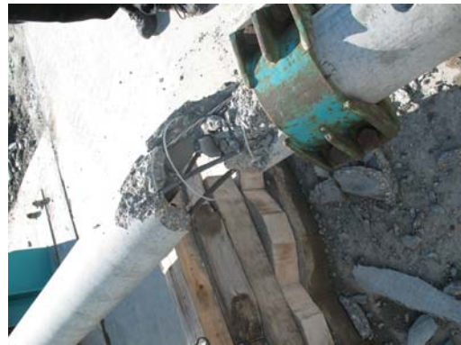
d) Failed collar section
