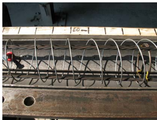
Figure 4.15: Spacing the helical reinforcing
