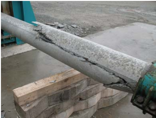
c) Cracking pattern (back side)
