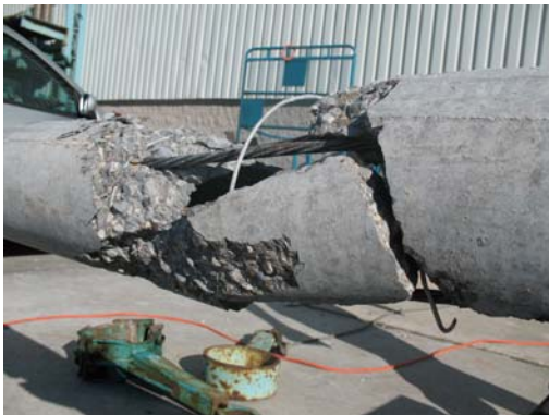
e) Failure at collar (loading side)
