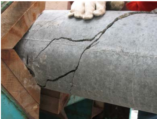
c) Crack pattern (back side)
