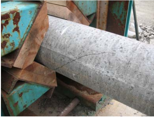
a) Initial cracking at butt
