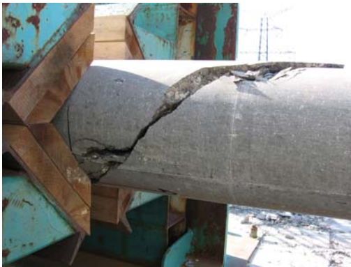
c) Failure pattern (back side)
