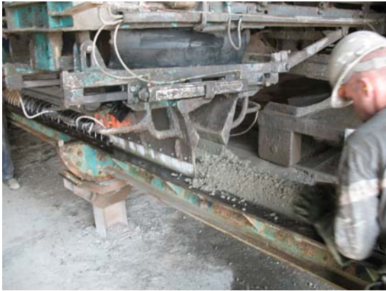
Figure 4.16: Pouring and placing of concrete
