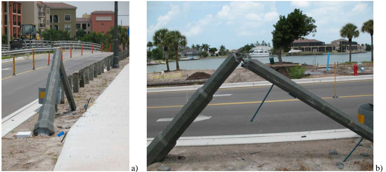
Figure 1.2 a) and b): Pole failure caused by vehicle impact and inertia effects (Sky Cast Inc., 2007)
