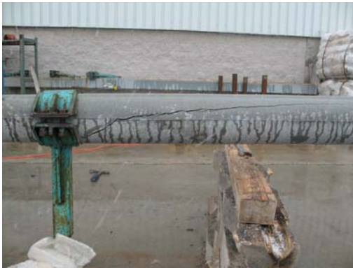
c) Cracking pattern (front side)
