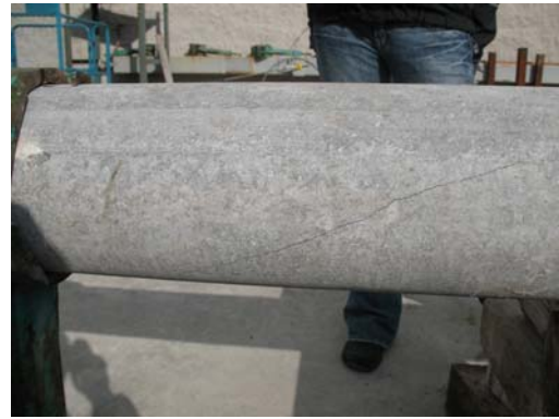
b) Cracking at loading collar (loading side)
