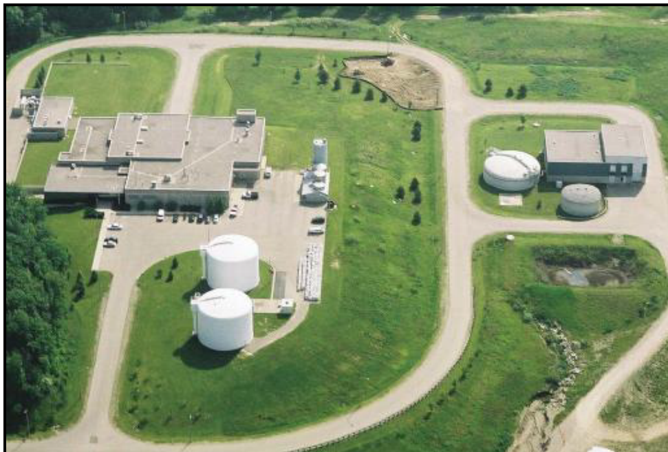
Figure 3.1: The Mannheim Water Treatment Plant in Kitchener, ON (Emelko et al. , 2006).
