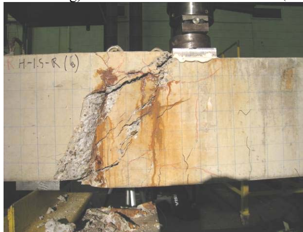
H(M)-1.5-R (Diagonal Crushing)
