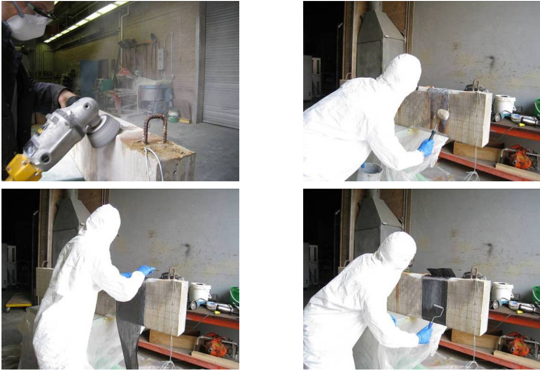
Figure 3.16 CFRP Application
