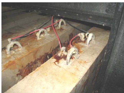
Figure 3.15 Anode and Cathode Connections
