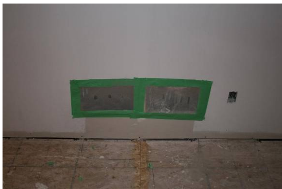
Figure 28 - Prototype House Return Air Cover Post Drywall
