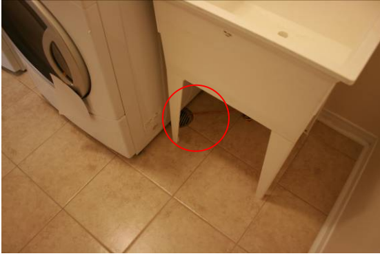
Laundry Room Tile with Drain
