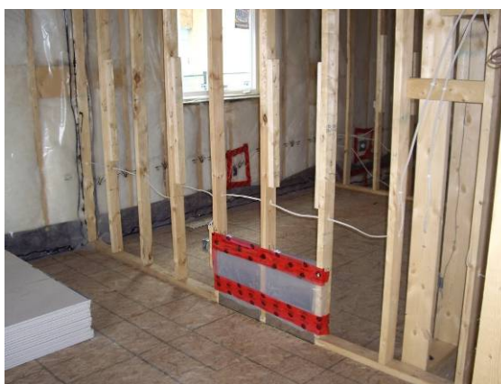
Figure 27- Prototype House Return Air Cover Pre-Drywall
