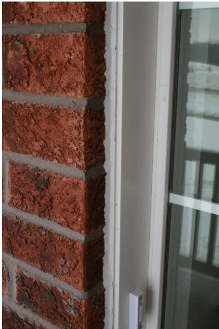
Caulked exterior Cracks/Openings
