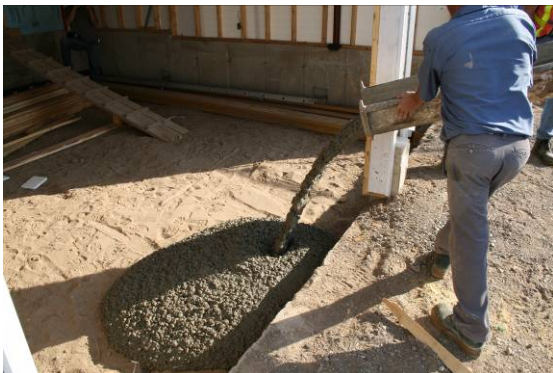
Leftover Concrete as Backfill
