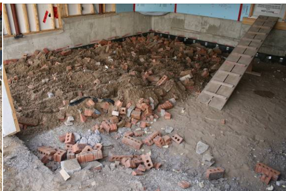
Leftover Brick as Backfill
