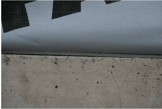
Wood to Concrete with Sill Gasket
