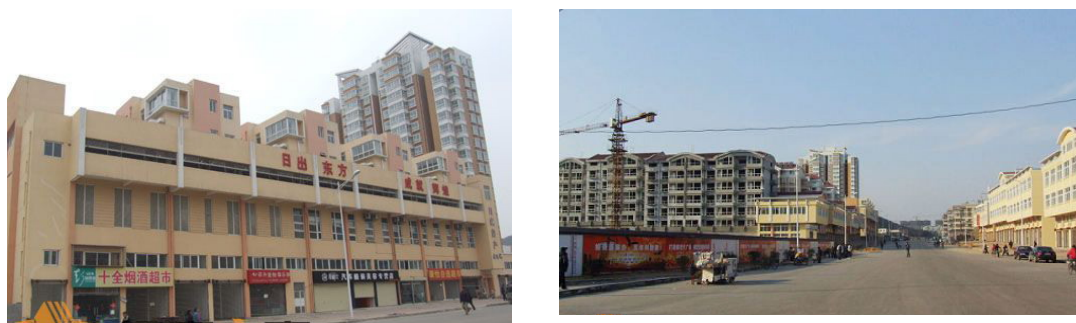
Figure 5.1 The Retail Stores in a Main Street in a Residential Community in Xuzhou
