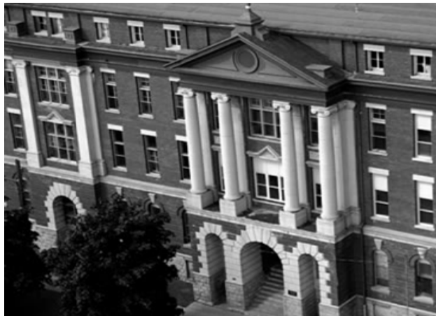
Figure 4: WLU Faculty of Social Work, downtown Kitchener
