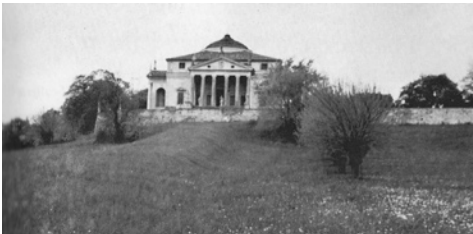
Fig2.2; Palladio's Villa Rotunda sits on a hill and overlooks all the land under ownership by the landlord.
