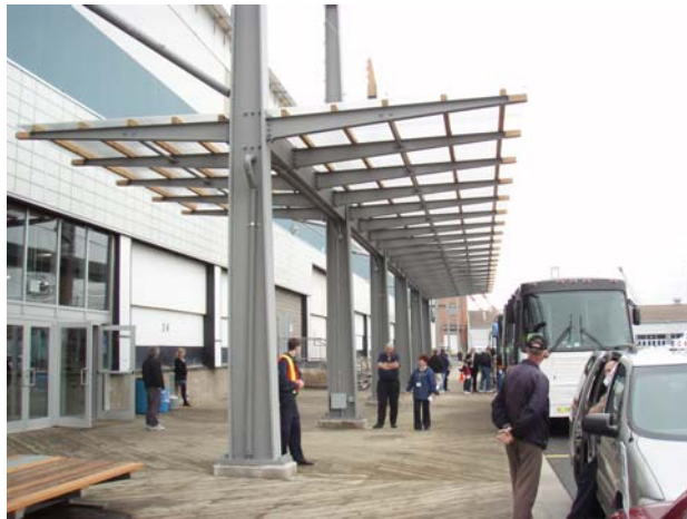
Figure 5.6: The Pier 22 Cruise Pavilion
