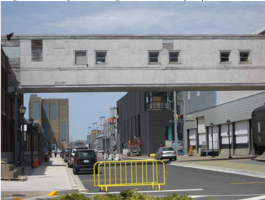
Figure 5.12: The View Leading Cruise Ship Visitors to the Rest of the Halifax Waterfront
