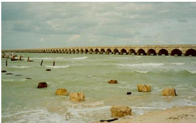
Figure 6: Stainless steel rebar was first used in Progreso Pier, Yucatan, Mexico (Arminox, 1999)
