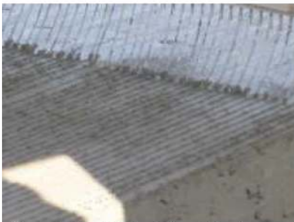
c) Longitudinal Tining (Close View)
