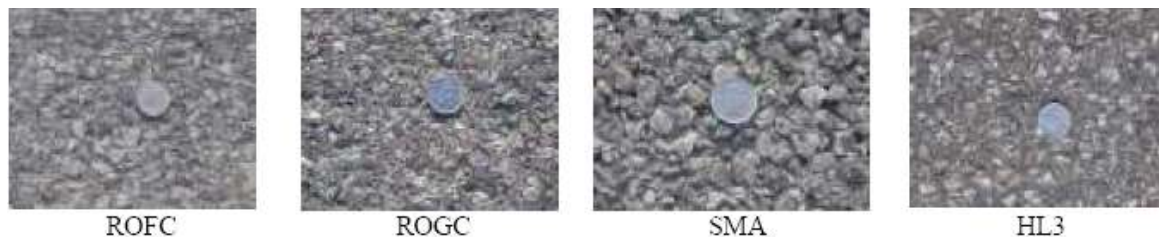
Figure 4-13 AC Pavement Surfaces at CAPTT-ROW Quiet Pavement Test Site.
