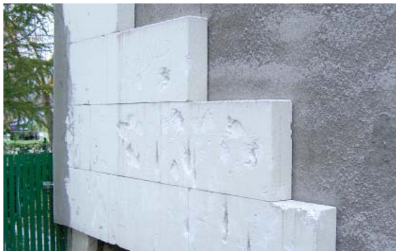
fig. 1.16 Warsaw, Wrzeciono estate, newly renovated tower.
