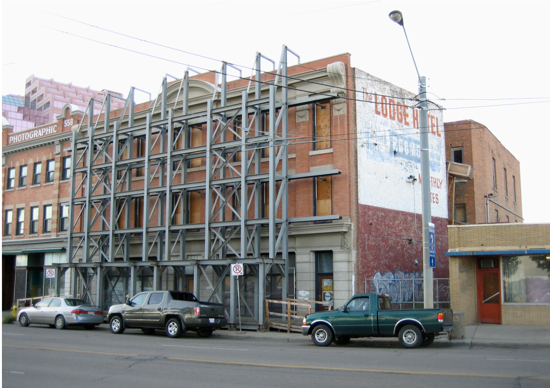
Figure 4.11 Lodge Hotel Under Construction in 2008
