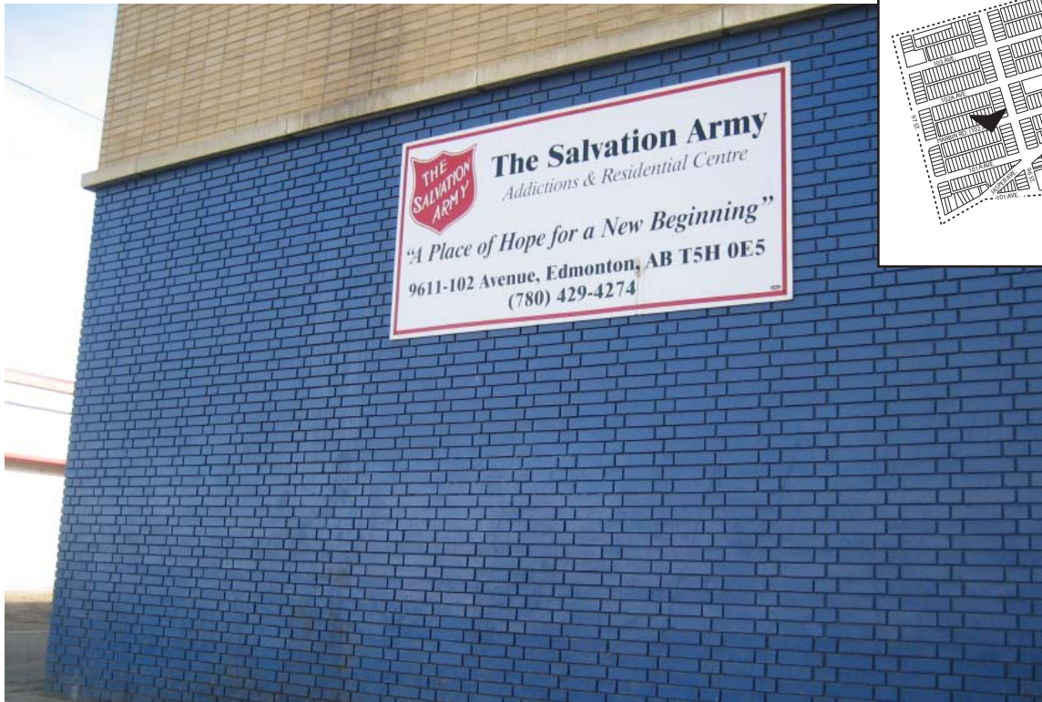
Blank facade of the Salvation Army's Addictions & Residential Centre
