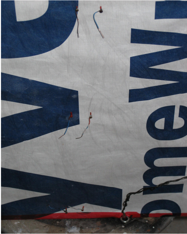
Figure 4-14: Three Pairs of Moisture Pins Installed in Tyvek covered OSB
