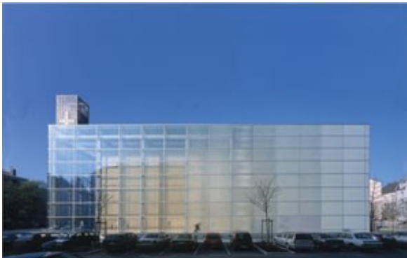
figure 4.5 elevation of Herz Jesu Church showing the transition in the opacity of the glass.
