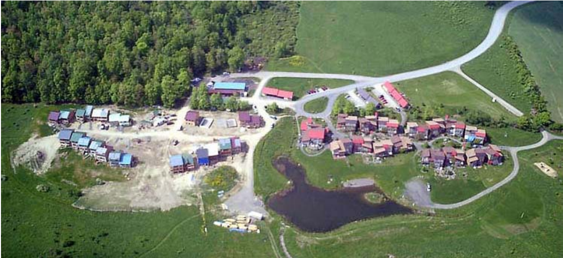
Figure2-27: Aerial view of Eco Village Ithaca in New York State, USA. Founded in 1991, the Ithaca Eco Village is a firm example of a successful self-sustainable community. Village residents all work where they live, and contribute to the use and maintenance of two 30-home co-housing neighbourhoods, FROG and SONG, and a third neighbourhood ( TREE ) in the planning stages, an organic CSA vegetable farm, an organic CSA/U-Pick berry farm, office spaces for cottage industry, a neighbourhood root cellar, community gardens and varied natural areas. Over 80% of the 175 acre site is planned to remain green space, including 55 acres in a conservation easement held by the Finger Lakes Land Trust. 26
