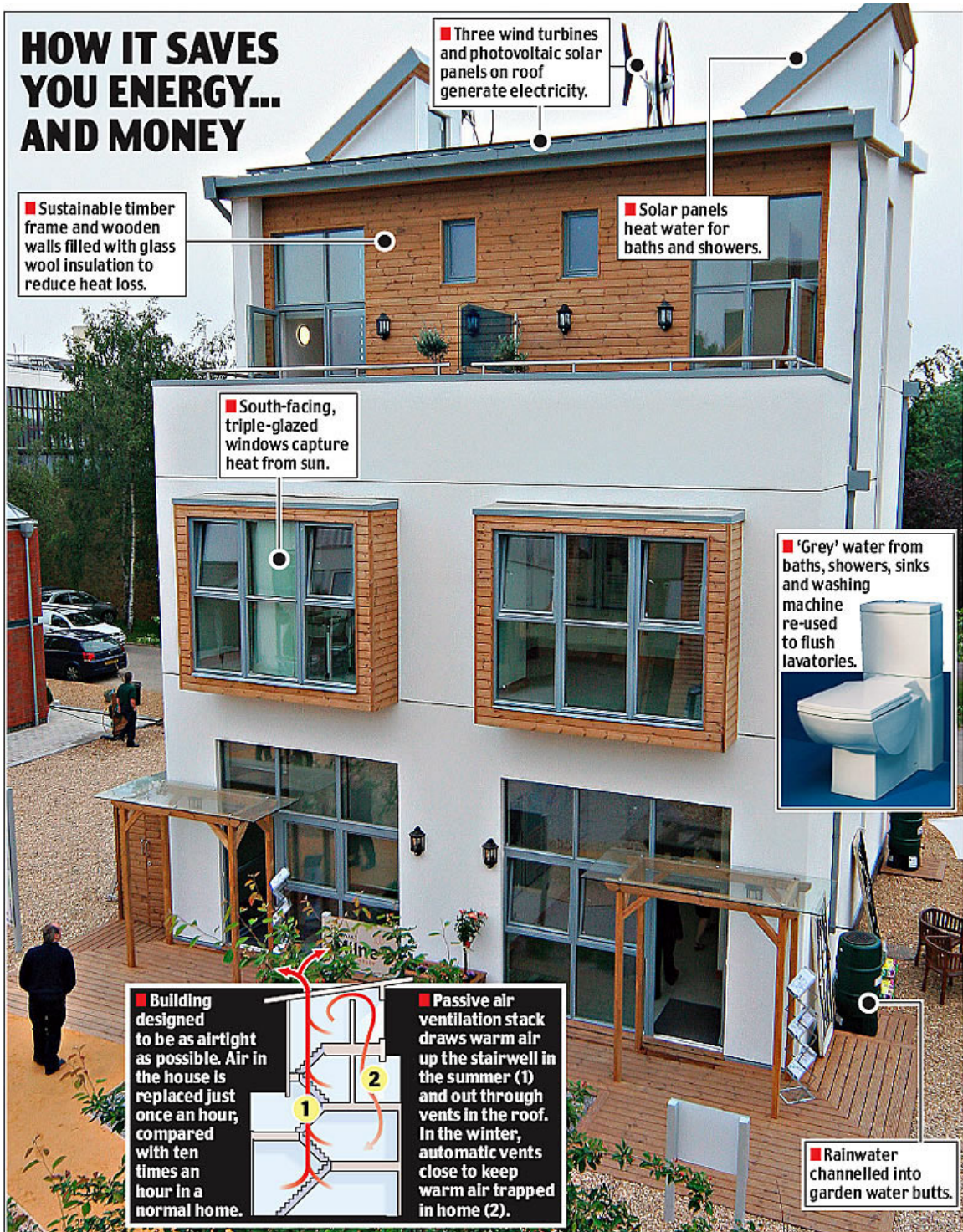
Figure 2-19: Diagram above briefly shows how the various systems for renewable energy work in a zero carbon house. Not only is this home in harmony with the natural world but it is also saving the owner a great deal of energy and money.
