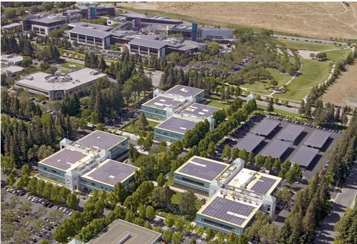
Figure 2-36: Photograph of the 1.9 MW solar electric project at the main Google headquarters in Mountain View, California. This project includes solar array designs for three different types of rooftops and two different steel carports. Solar power can be used in two different ways: 1) Solar panels or slates can convert the sun's energy to heat in order to provide hot water, or 2) Photovoltaic tiles can create electricity. Both types of solar power will not only save a building owner money, but will also significantly reduce the carbon emissions of the building.
