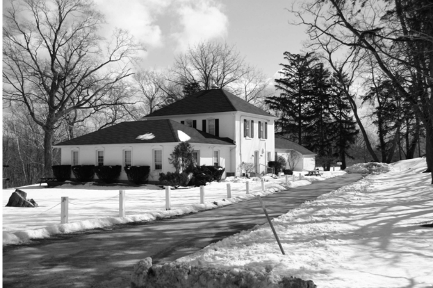
Figure 3-4: The first sign of architecture at the Burloak Employment Lands was this Farm house, built before the first oil refinery moved into the Burloak Employment Lands. The house now serves as a corporate meeting place for Petro-Canada business executives.
