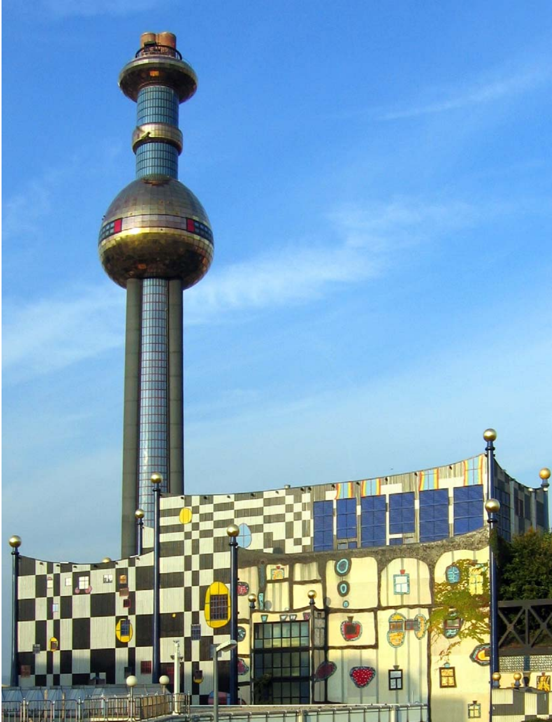
Figure 2-39: This incineration plant is one of several plants that provide district heating to the city of Vienna in Austria. Incineration is a popular Waste-to-energy technology generally used to create energy in the form of electricity or heat from a waste source. Such technologies reduce or eliminate waste that otherwise would be transferred to a landfill.
