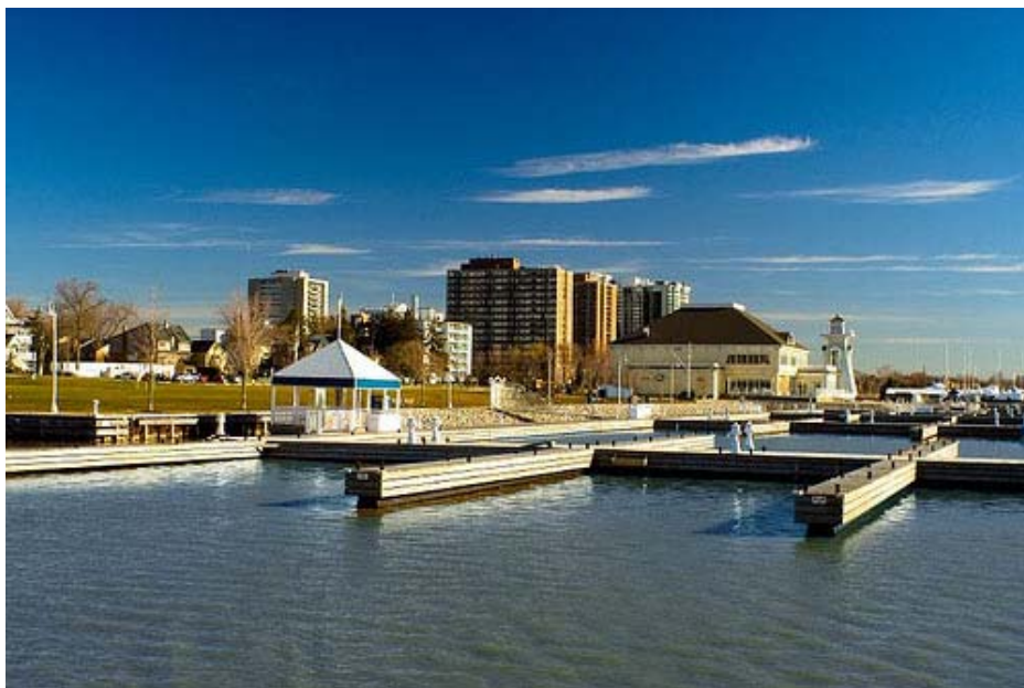
Figure 3-19: Photograph of the Bronte Village Harbour. The harbour houses a wide mix of activities and buildings, including apartment buildings, restaurants, shops, and recreational parks facing the water.
