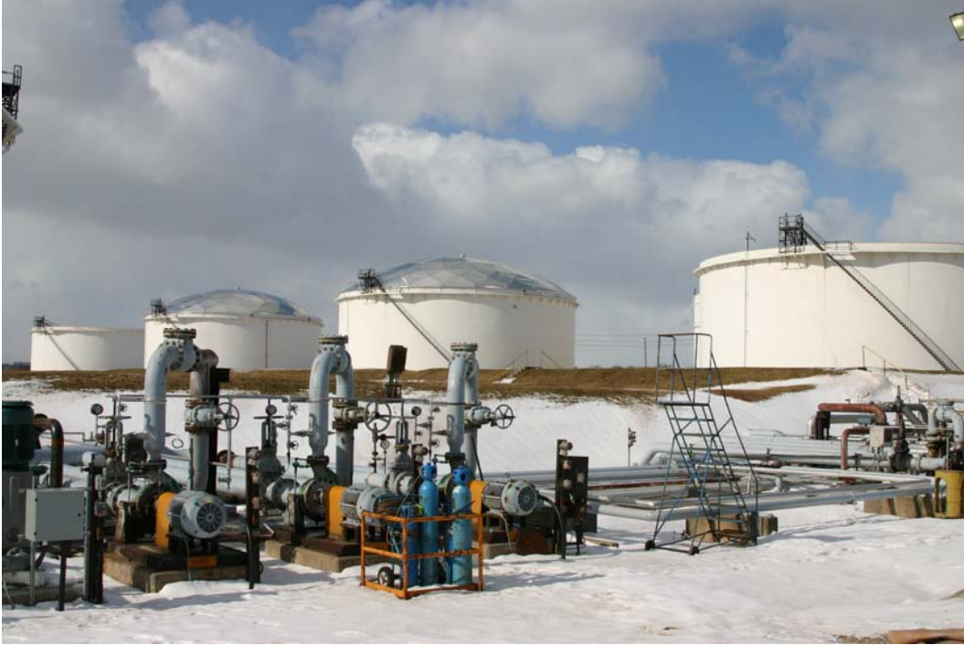
Figure 3-10: Ethanol Domes are similar in scale to gasoline tanks but require a dome ceiling.
