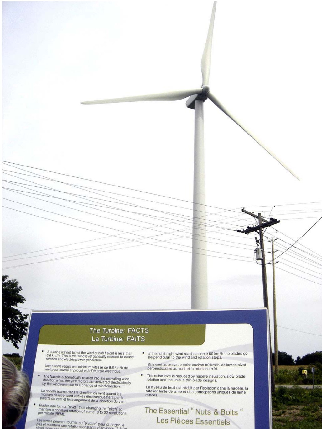
Figure 2-37: Photograph of one of the windmills at the Erie Shores Wind Project in Southern Ontario. The project brings 99 Megawatts of electricity into Ontario Hydro’s main power lines. Due to the fact that wind is inconsistent, the wind turbine project cannot be used as a primary source of power, however, wind power can significantly reduce the stress on conventional means of generating electricity. Out of the 550 Kv of electricity generated by Ontario’s main power plants, 115Kv are generated by wind power. Each wind turbine in the Erie Shore Wind Project cost approx. $2million dollars and generates 660 Volts of electricity (Enough to power approx. 700 homes). There are 66 wind turbines in total spread across several farms in Southern Ontario. The sites were identified by research studies as strategic places to locate wind turbines.
