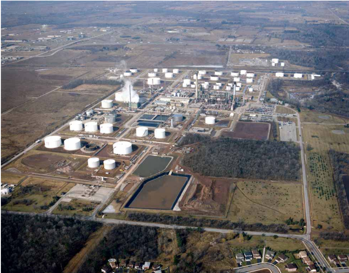
Figure 3-6: Aerial photograph of the Petro Canada Plant in Oakville back in 1986.
