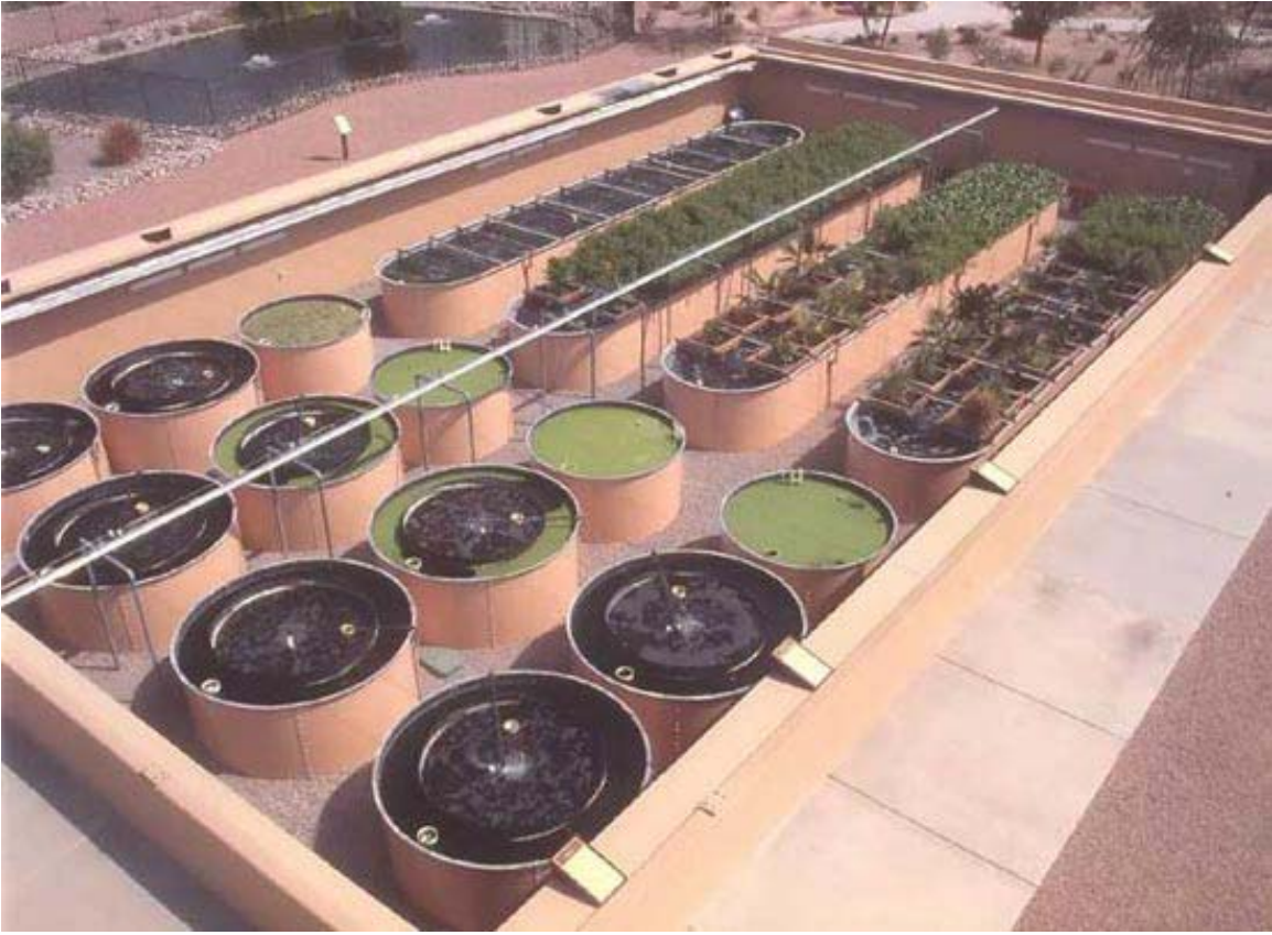
Figure 2-35: Photograph of a Living Machine System invented by biologist John Todd as an engineered solution to managing human and manufacturing wastes in today's water systems. Living Machines are natural wastewater treatment systems, site-specifically engineered to imitate the water-cleansing properties of natural wetlands (i.e. ponds, marshes and meadows). Unlike septic and other chemical treatment systems, the technology relies entirely on living organisms to convert "wastes" into healthy nutrients. Water treated by Living Machine technology is currently being reused around the world for irrigation, indoor plumbing, and more.
