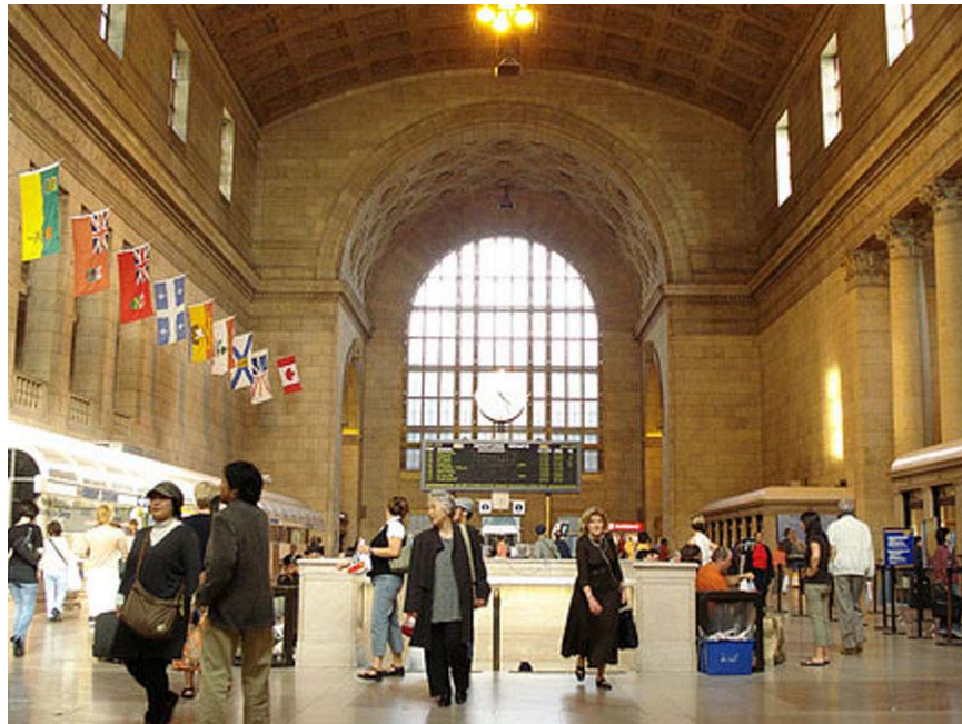
Figure 2-14: Completed in 1927, Union Station in Toronto is an excellent example of a pre WWII building that has withstood the test of time. Its solid “skin” or building enclosure serves as structure, insulation and finish all in one thick masonry layer. Unlike many of the buildings constructed after the war, the exterior shell of Union Station is practically intact and likely to last at least another 100 years.
