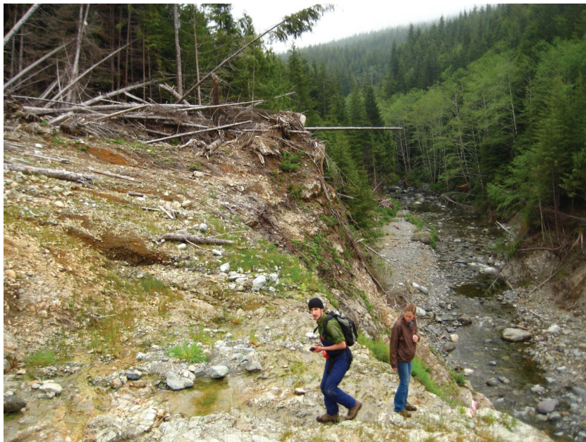
Figure 4.13. A dramatic example of a stream removing landslide deposits is shown here at the toe of a landslide on Vancouver Island.
