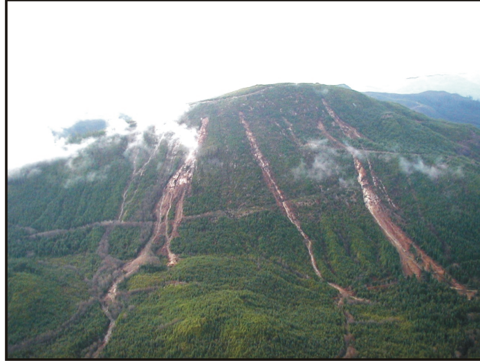
Figure 3.3. An example of landslides following the 2001 storm in Loughborough Inlet (Guthrie and Evans, 2004b)
