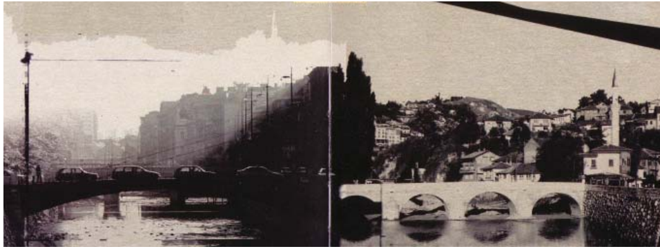
Fig. 3.15: Novi Most Bridge and Šeher Ćehajina Ćuprija Bridge
