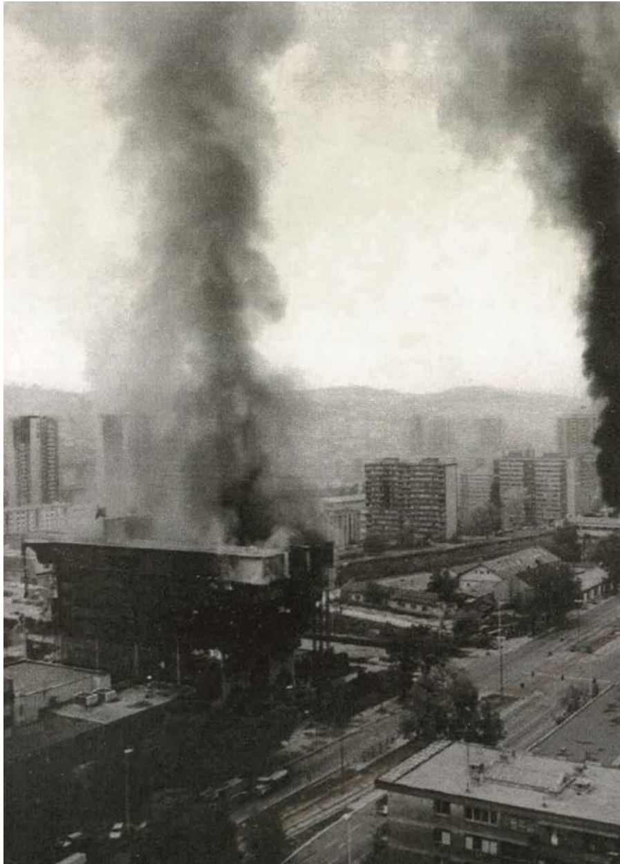
Fig. 3.8: Destruction of Electropivreda building
