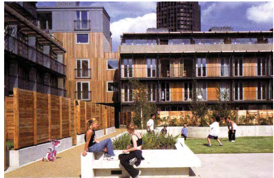
FIG A.24 Photo of Interior Courtyard
