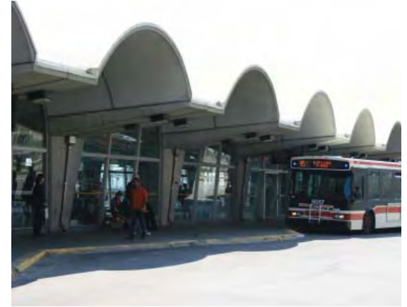
3 - kipling subway station
