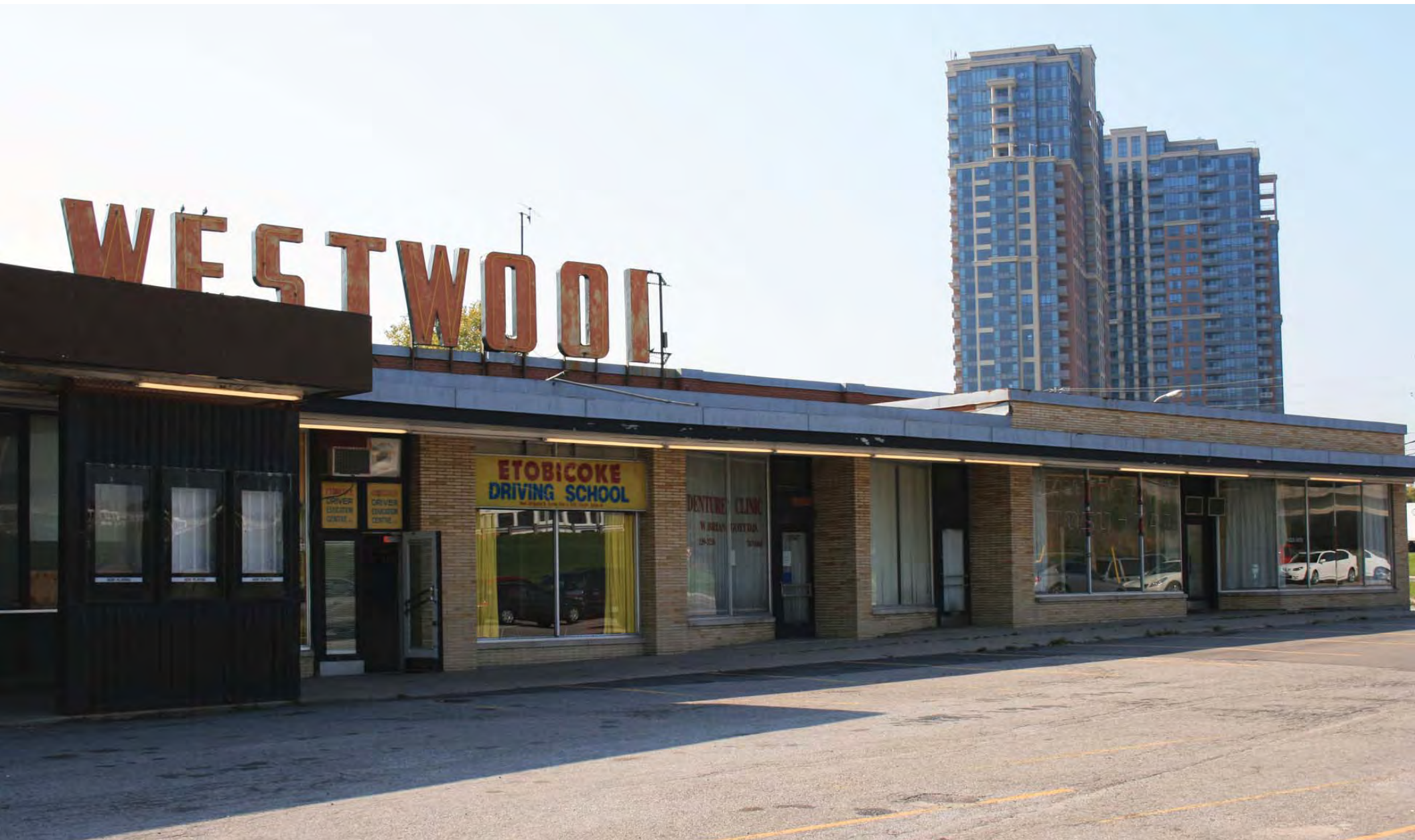
FIG 4.13 Photo of the former Westwood Theatre
