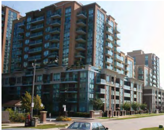
5 - mid-rise podium apartment building
