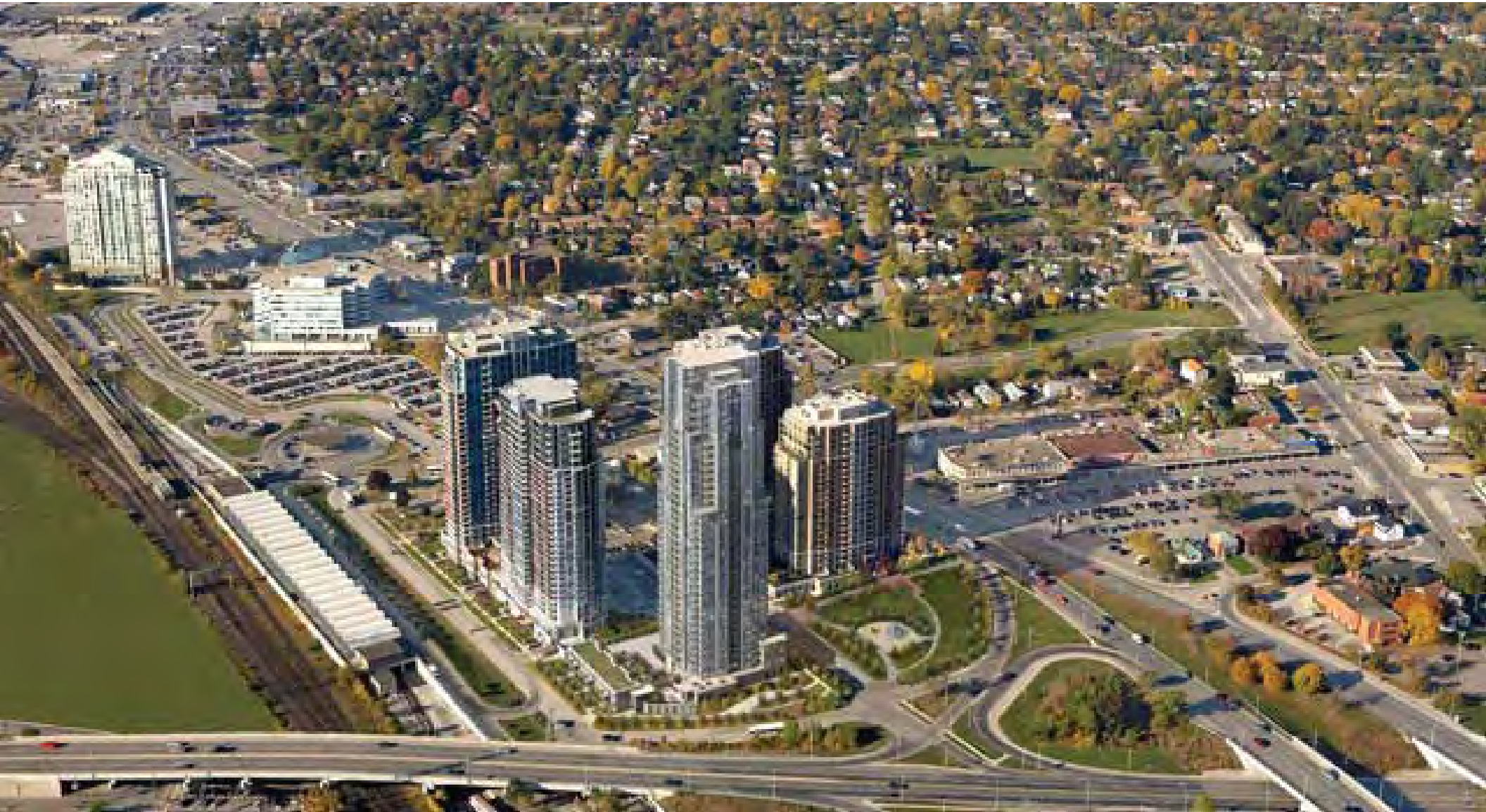
FIG 4.06 Tridel Development Site, immediately adjacent to Kipling station
