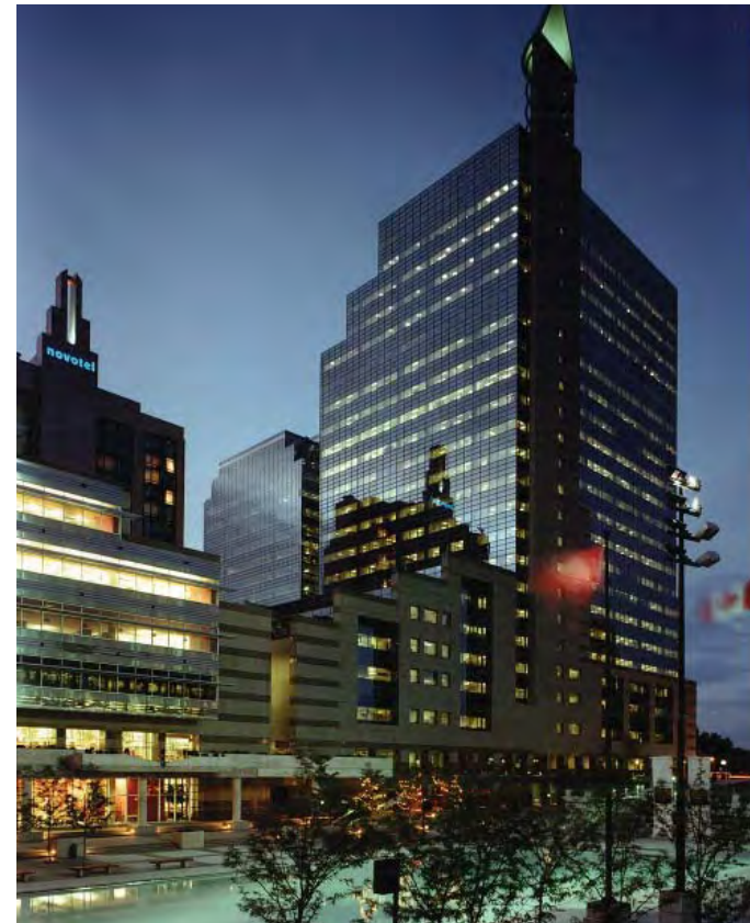
FIG 1.12 Suburban downtown in North York started with the building of North York Civic Centre.
