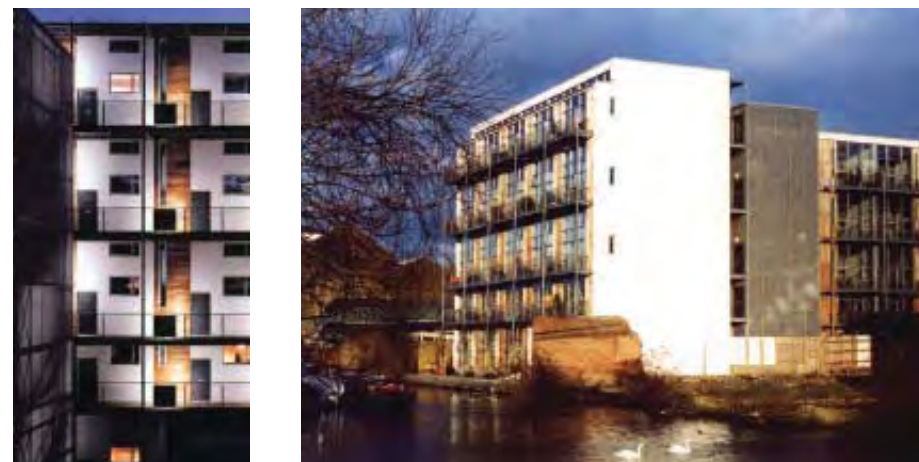
FIG A.28 Photos of Interior Courtyard and view from canal
