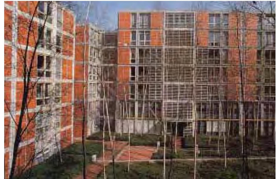
FIG A.30 Photo of Interior Courtyard
