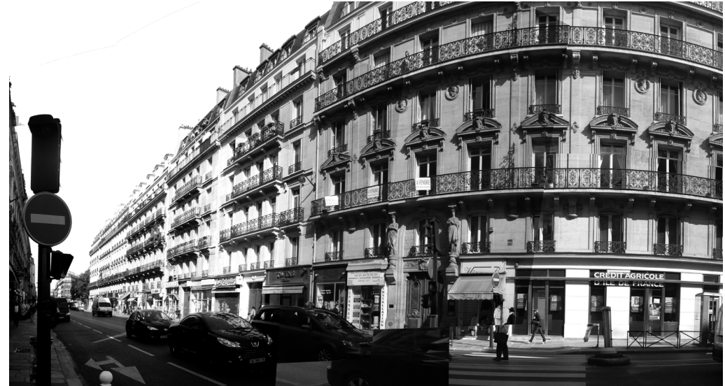
4.4 Metro Poissonnière and the 19th century façade along Lafayette
