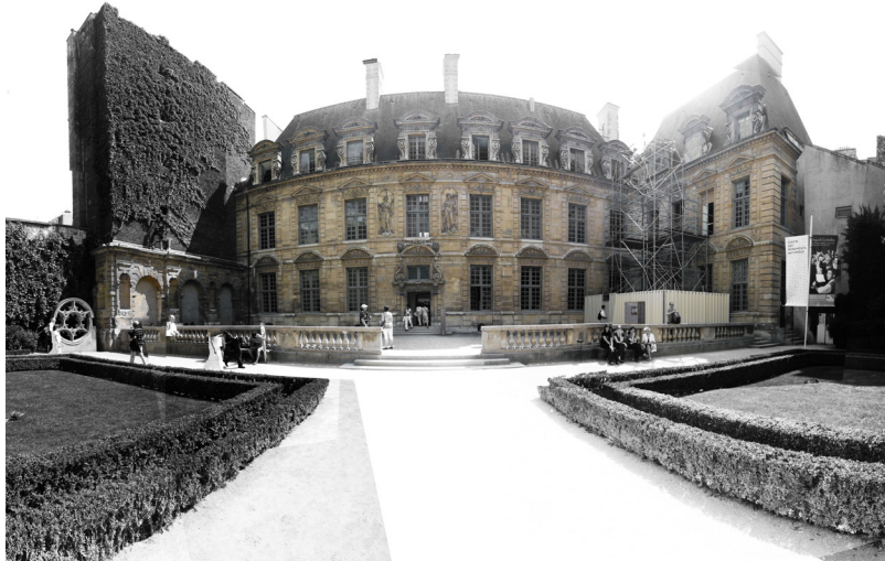
2.13 garden façade of the hotel Sully
