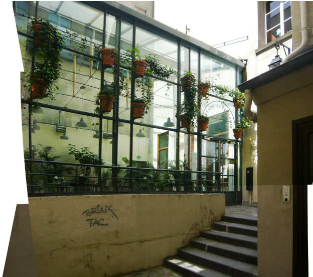
6.5 Tertiary courtyard in St. Paul's Village, Paris 4eme Arrondissement
