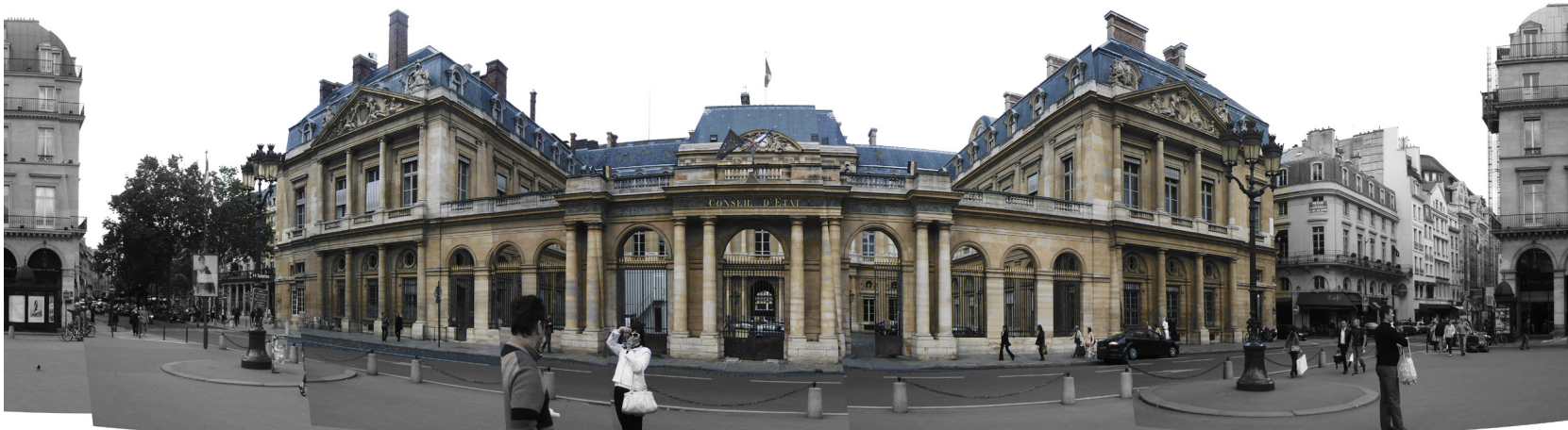
1.8 Street façade of Palais Royale in 2009. Originally called Palais Cardinal.
