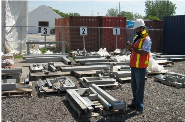
Figure 3.9 – Worker using a mobile RFID reader in a construction laydown yard
