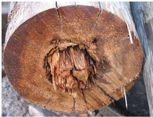
(a) Decay at the centre of the pole section
