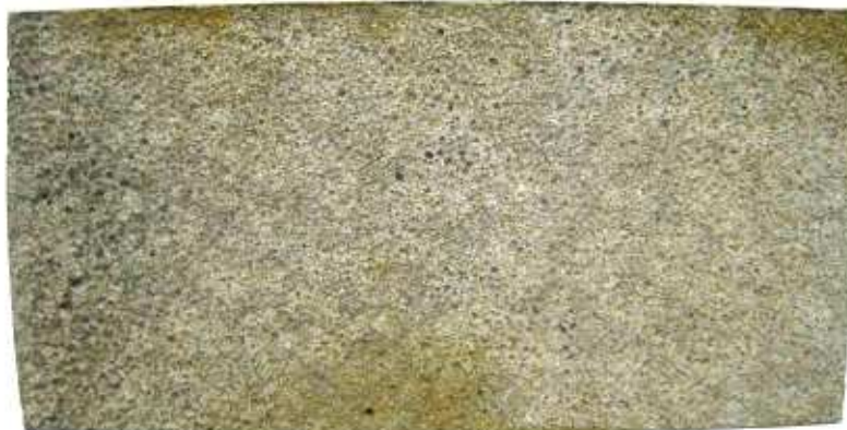
Figure 3.13: Pickled specimen with heavy corrosion (old steel)
