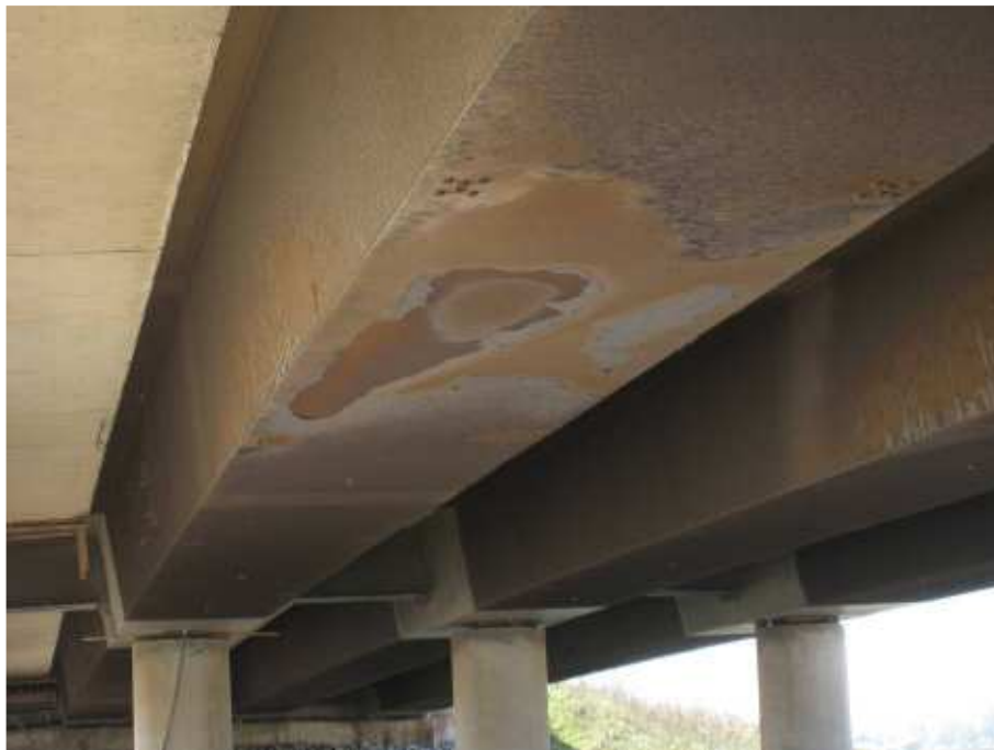
Figure 1.1: Underside of highway structure
