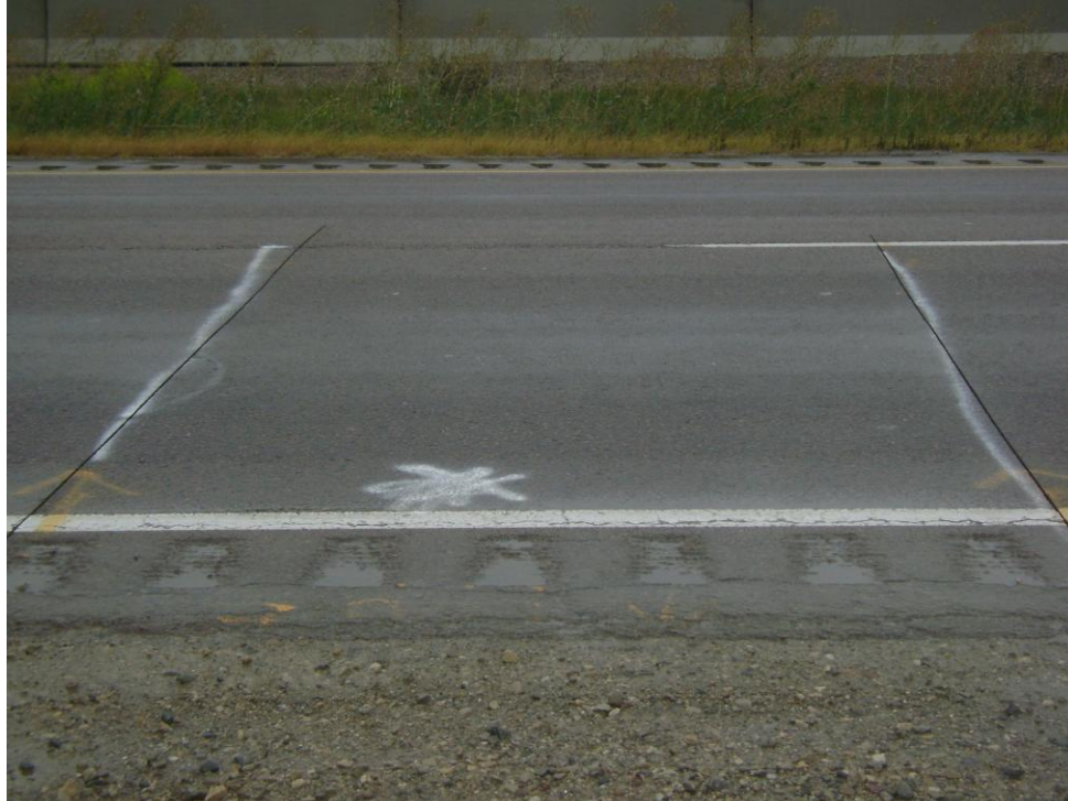
Figure 3-19: Pavement Marking Prior to Open Trench Excavation
