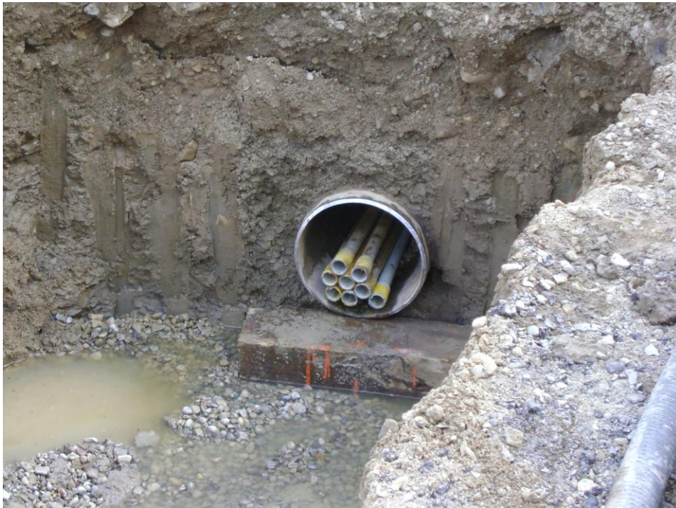
Figure 3-21: PVC Tubes Inside the Steel Conduit
