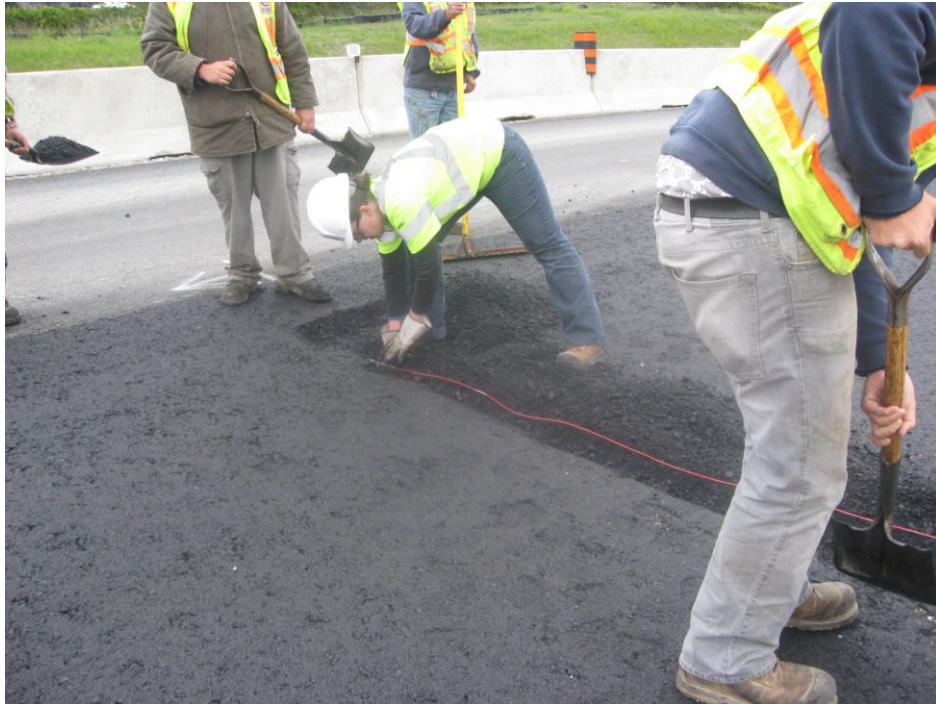
Figure 3-25: Placement of Strain Gauge and Covering the Wire Trench
