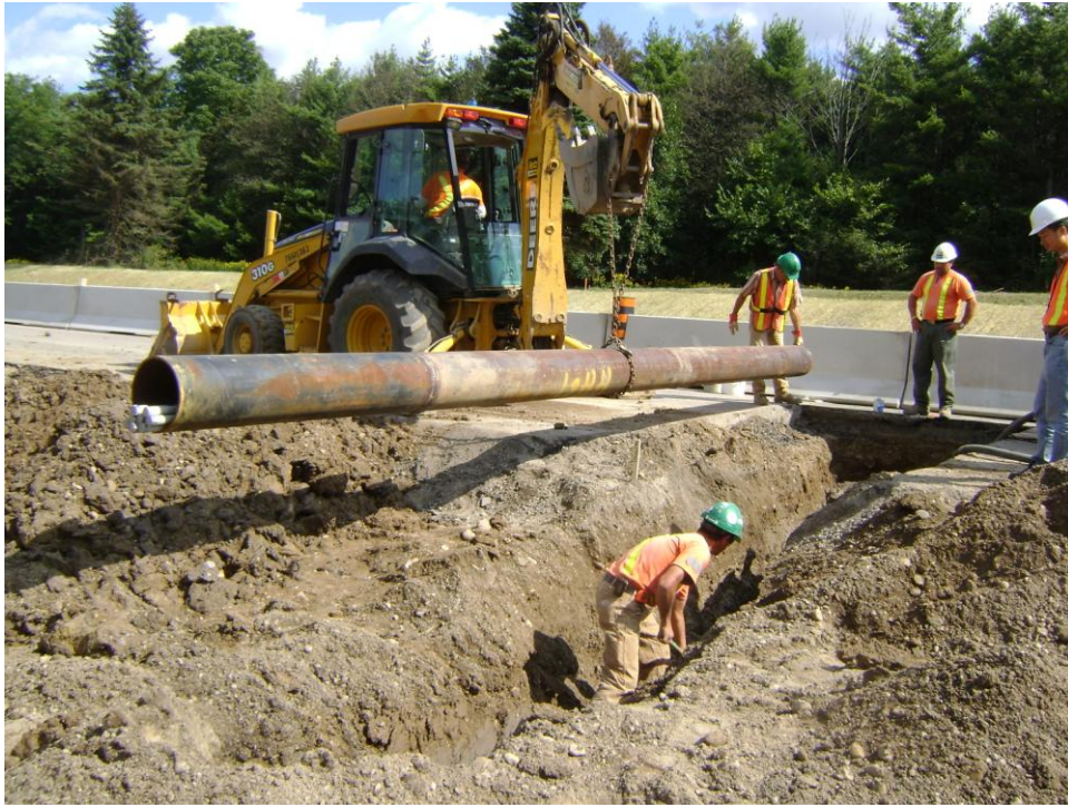
Figure 3-20: Conduit Installation
