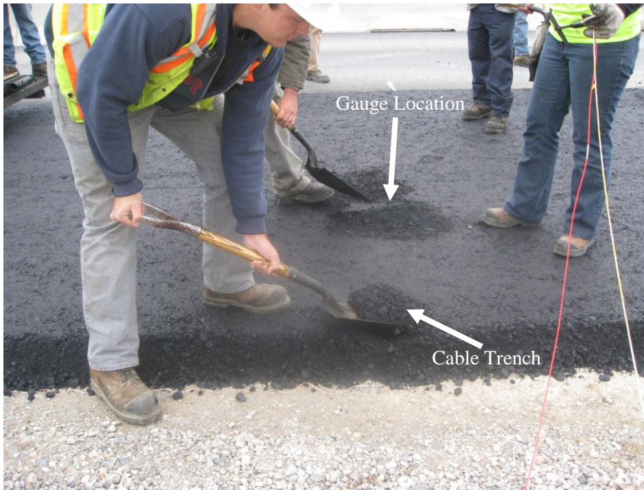
Figure 3-24: Removing Asphalt Material to Place the Strain Gauge at Bottom of the Layer
