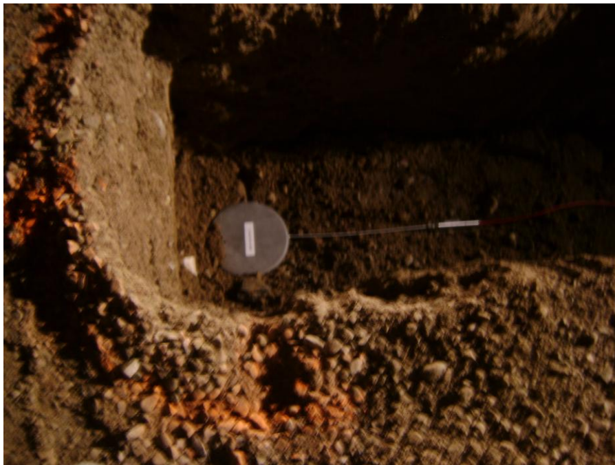
Figure 3-27: Installation of Earth Pressure Cell
