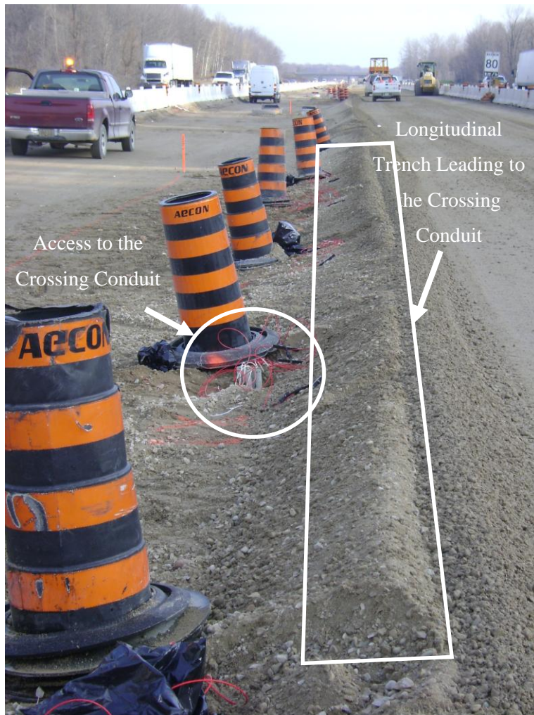
Figure 3-22: Pre-Installation Site Preparations
