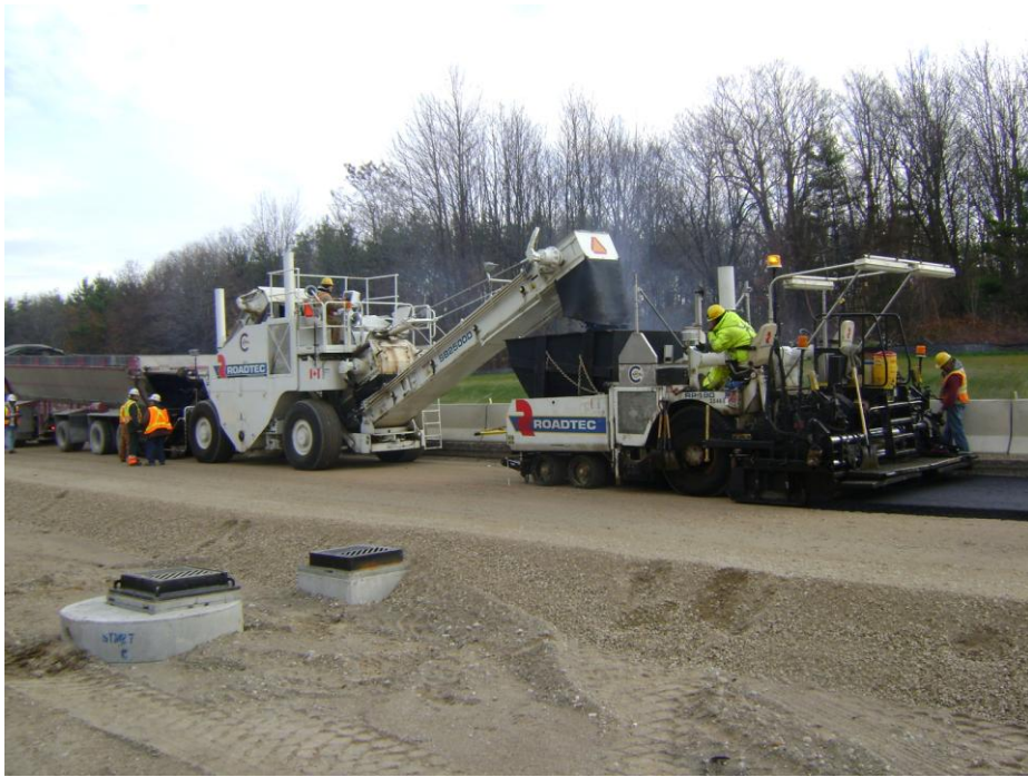
Figure 3-23: Asphalt Paver and Shuttle Buggy
