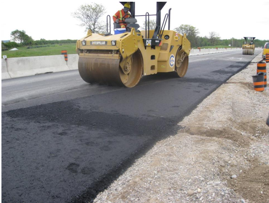
Figure 3-26: Monitoring Station after Strain Gauge Installation and Before Compaction
