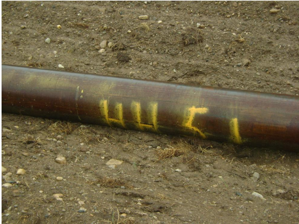
Figure 3-18: Steel Conduit Before Installation
