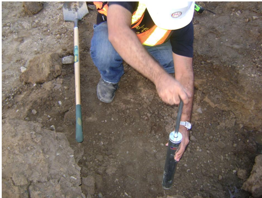
Figure 3-28: Compaction of Subgrade Surface Prior to Moisture Probe Installation
