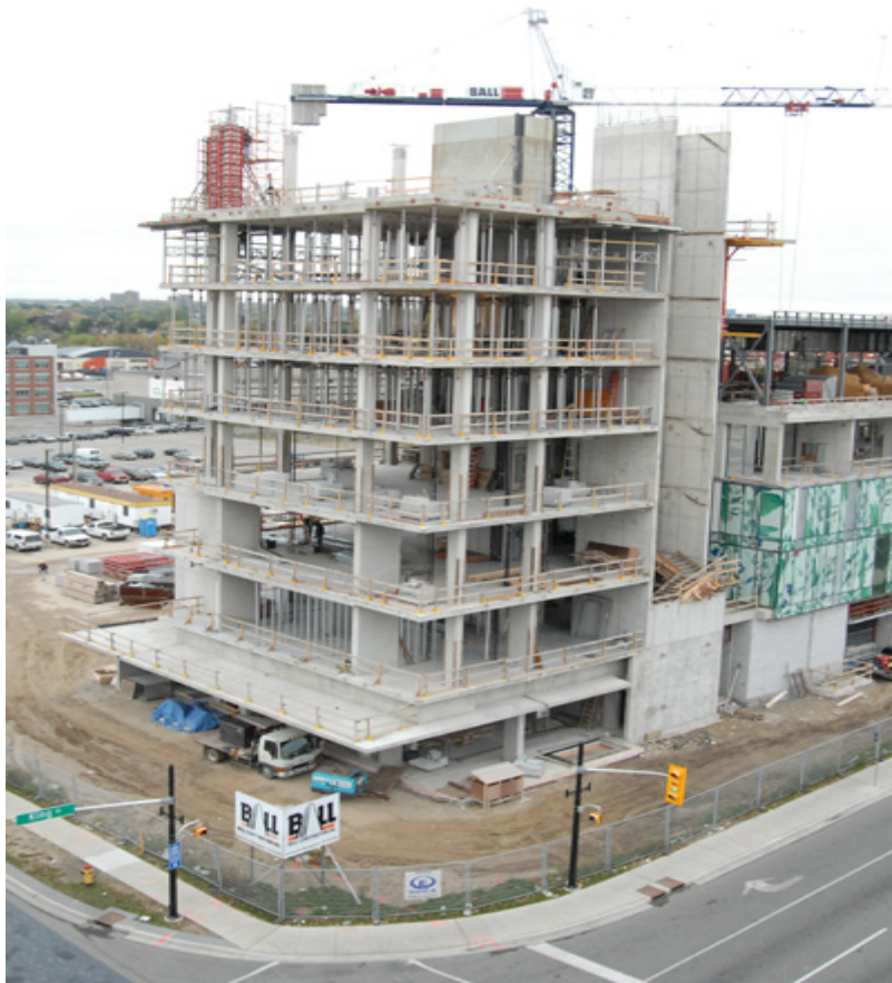
Figure 7.16: The UW School of Pharmacy under Construction
