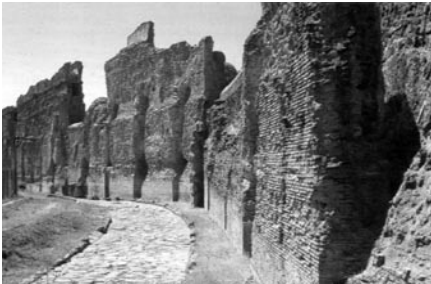
fig.4.47 RESTORED ANCIENT ROAD ( looking south)
