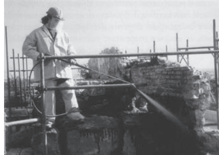
fig.4.43 WATER PRESSURE CLEANING OF THE AQUEDUCT
