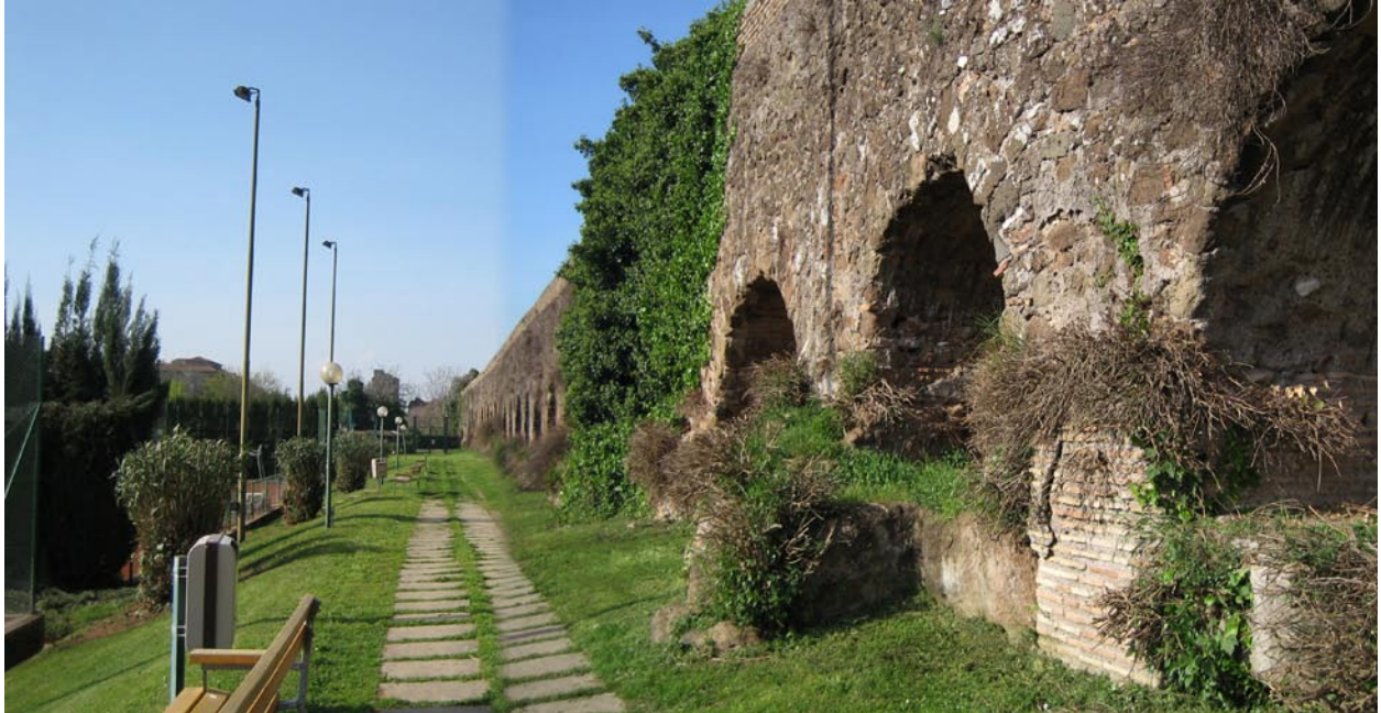
fig.6.25 PATH ALONG WEST SIDE OF ACQUEDOTTO FELICE (looking north)
