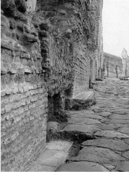
fig.4.46 DETAIL OF RESTORED ANCIENT ROAD ALONG THE AQUEDUCTS
