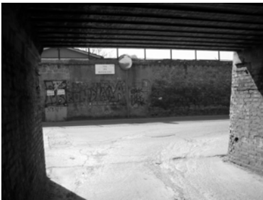
fig.7.41 UNDERPASSAGE (interior view looking out toward via del Mandrone)
