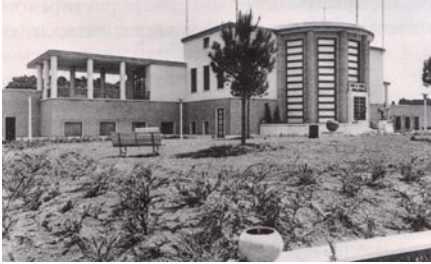
fig.4.17 'CLUB HOUSE' - EXTERIOR
