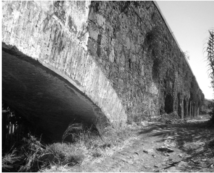
ACQUEDOTTO FELICE - DETAIL AT GROUND LEVEL fig.1.11 Wednesday, September 5th, 2007
