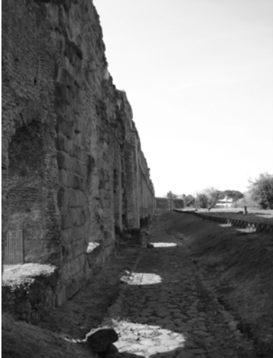
fig.7.19 ANCIENT ROAD ALONG AQUEDUCTS
