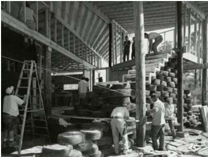
fig. 2.8 Students Building the Shiles House
