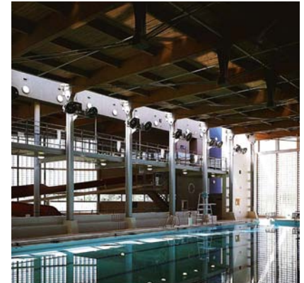
fig. 3.20 Milton Leisure Centre, Milton, ON
