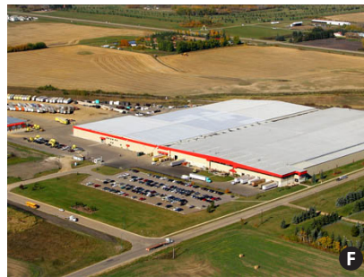
fig. 1.44 Home Hardware Distribution Centre
