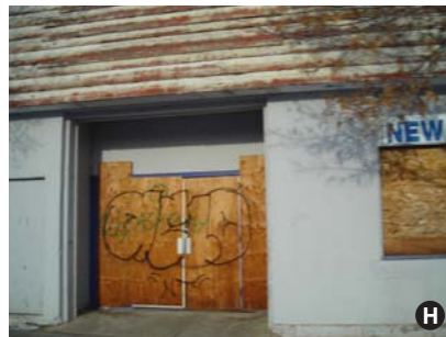
fig. 1.82 Vacant Building Downtown
