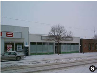
fig. 1.36 Downtown - Vacant Buildings
