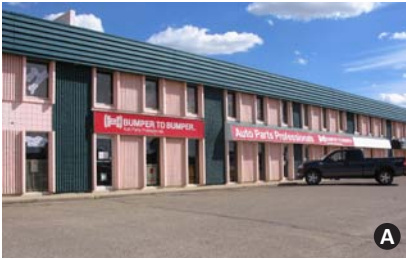
fig. 1.30 Highway - Strip Mall
