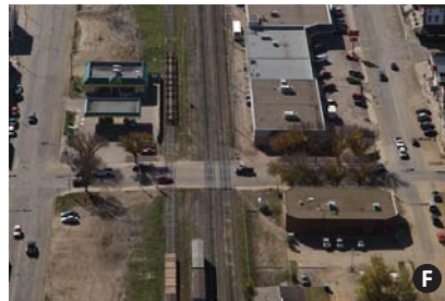
fig. 1.53 Railway crossing at Main Street
