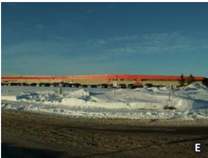
fig. 1.43 Home Hardware Distribution Centre
