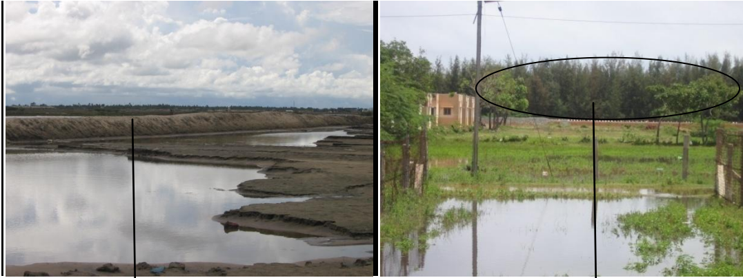
(a) Embankment created to prevent sea water from entering communities (Source: Field work) (b) Cashew trees planted along the coastline to protect communities from tidal waves (Source: field work)
