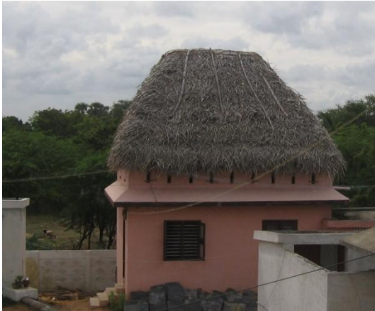
(a) Use of Thatch as a traditional element in design fenced houses (Source: Author)
