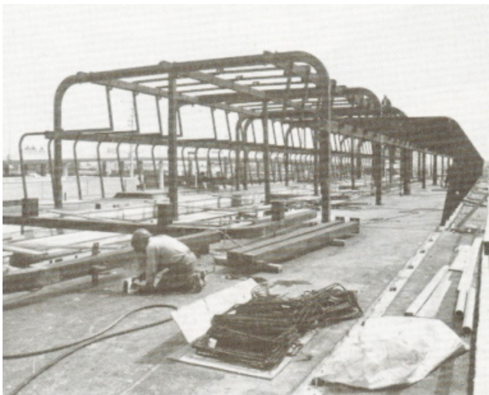
Fig 4.9 Aerial photo of Kennedy Station after opening in 1985 and photo of the steel framework of the SRT
