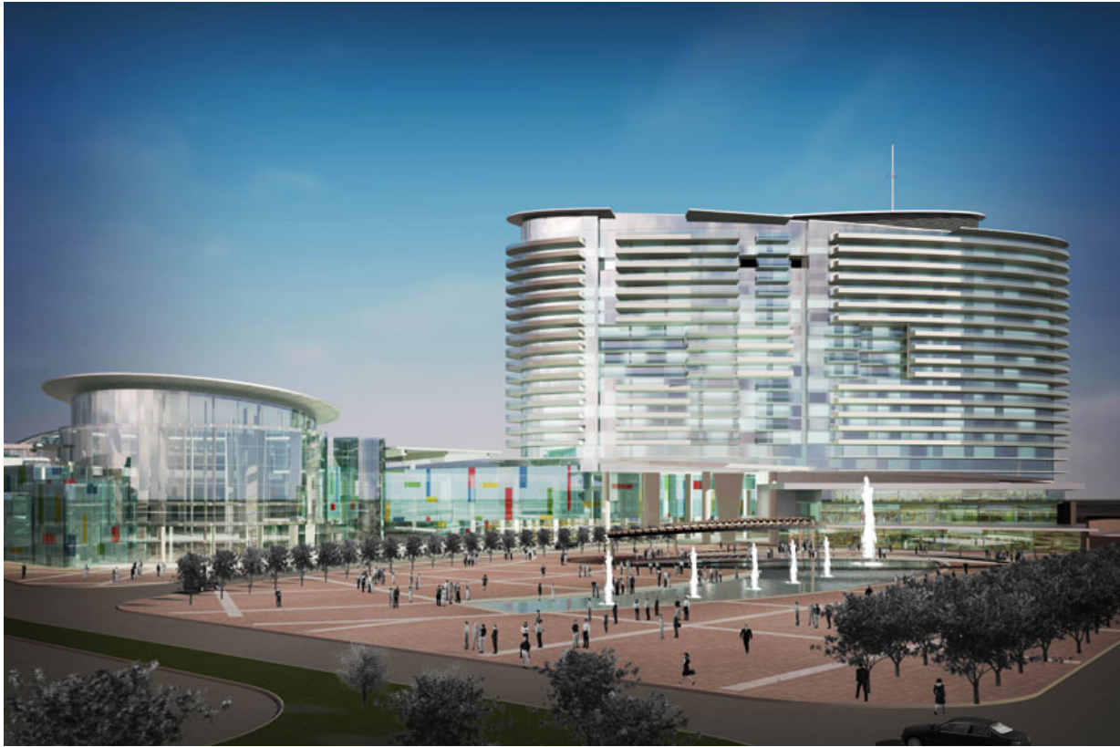
Fig 2.18 Remington Centre proposal for the redevelopment of Market Village in Markham, Ontario
