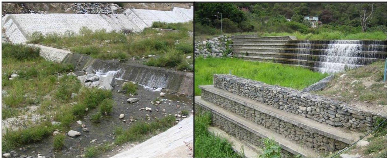
Figure 22: Sedimentation in Dams and Channels in 2008
