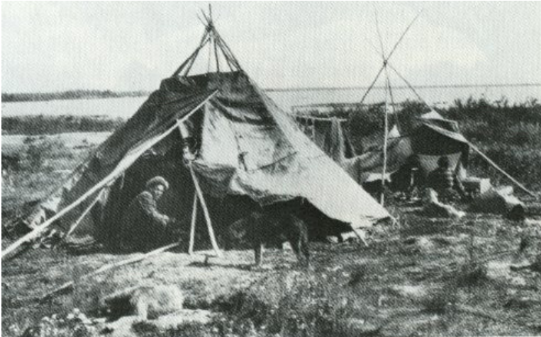
FIG.6.1. Caribou tepee, Fort Rae, 1913, demonstrates a traditional building typology for the region. Although contact has occurred at this point, traditional architecture remained unchanged. Simple in appearance, this structure had been modified through countless generations to suit the users needs to perfection.
