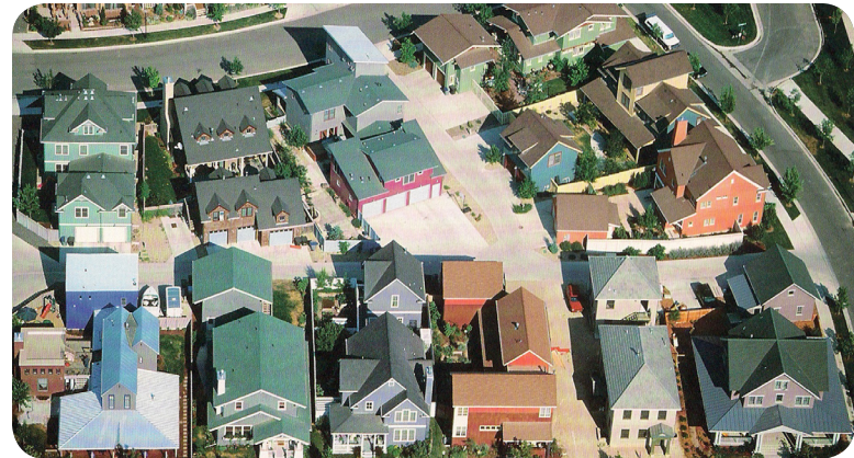
2.04 accessory units over residential garages in Longmont, Colorado
