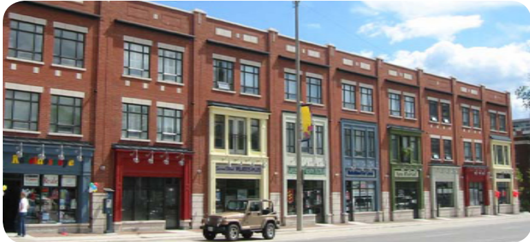
1.26 live work development in Port Credit, Mississauga, ON
