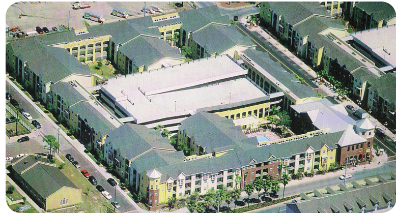
2.16 internal parking structure in Tampa, Florida
