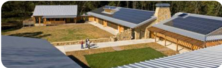
1.22 sustainable buildings with photovoltaic roof system
