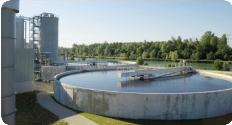
1.10 water treatment facility
