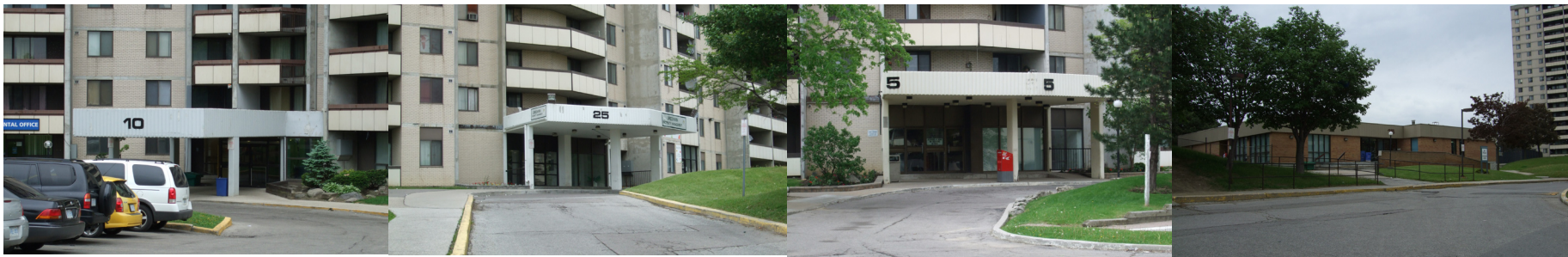
Fig 35. Building approaches from San Romanoway Boulevard
