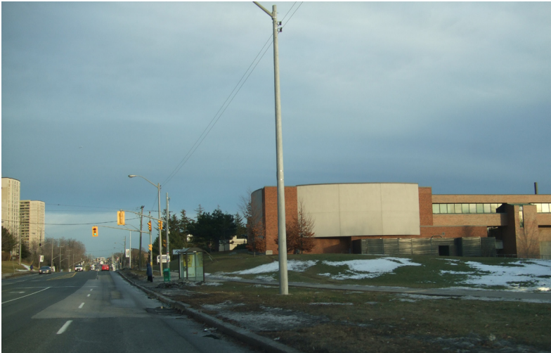
Fig 83. Street presence of Yorkwoods library theatre
