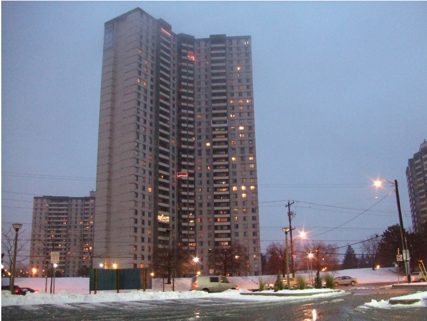
Fig 1. Palisades Apartment Complex Winter 2008.
