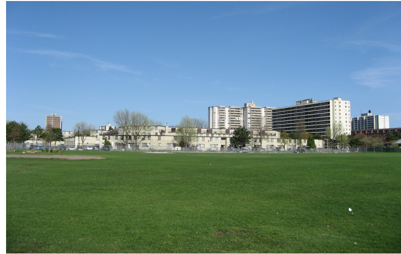
Fig 80. Approach to Connections from Flemington Park
