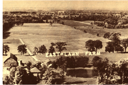
"...Jane/Finch was once a small farming district north of the City of Toronto. For nearly 150 years farms and orchards dotted the landscape ..."
