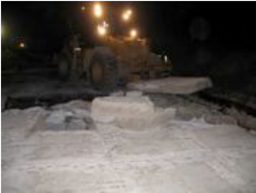
Figure 5.8 Removal of Waste Concrete
