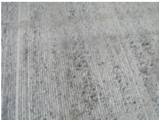
Figure 7.2 Pavement Surface Tining Close-up
