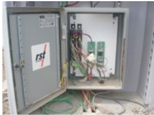
Figure 5.25 Relocated Multiplexers and Datalogger, and Wiring
