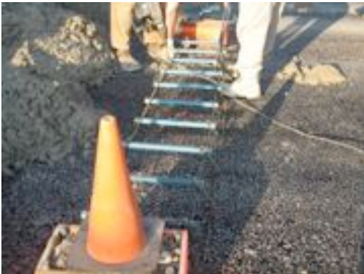
Figure 5.23 Inter-panel Extensometer Blockout Before Paving
