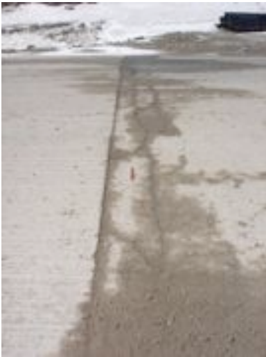
Figure 7.8 Asphalt Adjoining Test Sections
