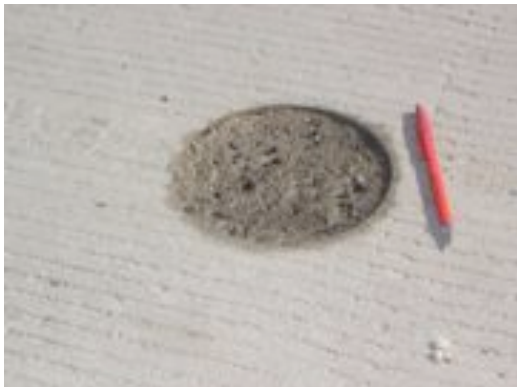
Figure 7.6 Core Hole Settlement
