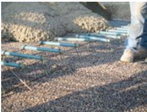
Figure 5.5 Skewing of the Dowel Bars
