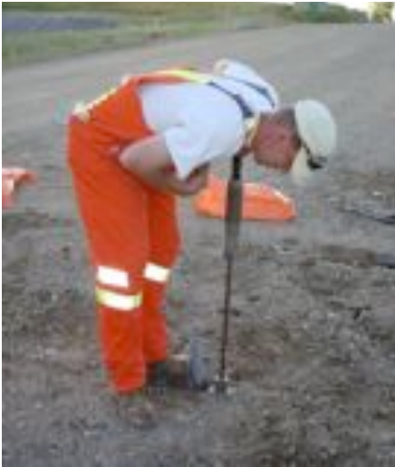
Figure 5.2 Marshall Hammer Compaction Around Sensor Conduit
