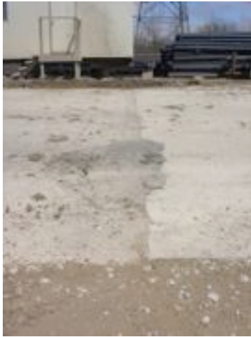
Figure 7.15 Patching of Adjoining Asphalt
