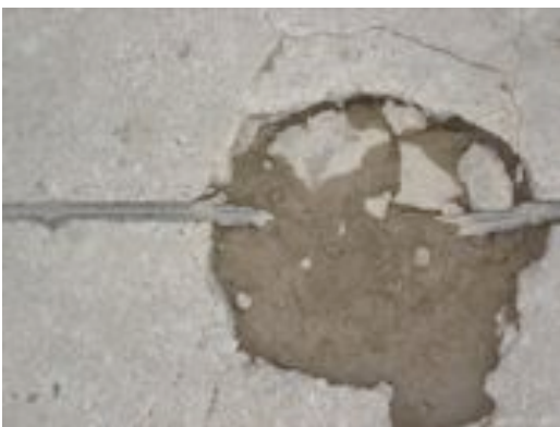
Figure 7.9 Blockout Failure
