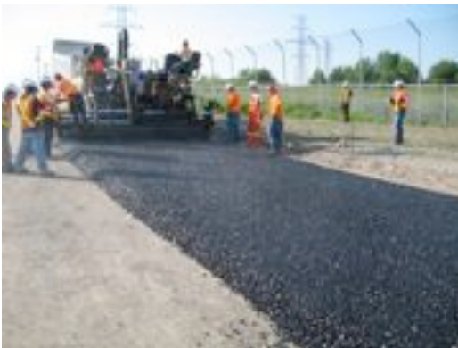
Figure 5.3 Paving and Compaction of ODGL
