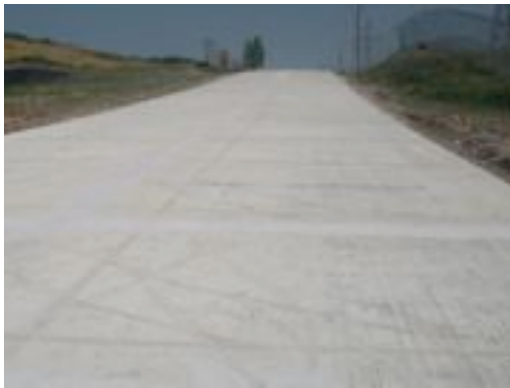
Figure 7.1 0% Coarse RCA Northbound View and 50% Coarse RCA Southbound View
