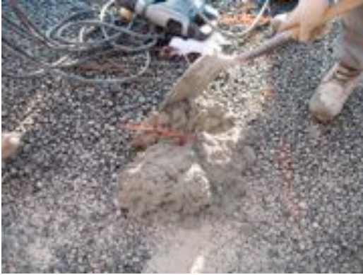
Figure 5.21 Mounding the Vertical Extensometer with Concrete
