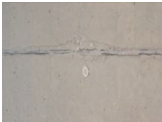
Figure 7.3 Joint Spalling
