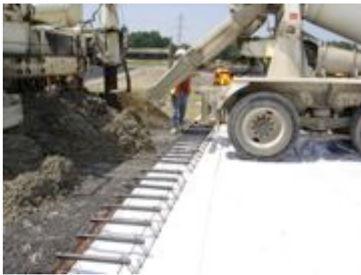
Figure 5.7 Placing Concrete for Removal
