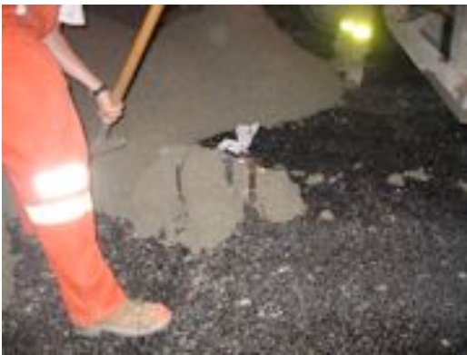
Figure 5.22 Mounding the Stain Gauges and Maturity Sensors with Concrete
