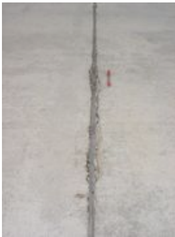
Figure 7.11 Joint Spalling
