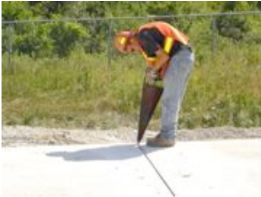
Figure 5.17 Widening and Sealing the Initial Saw Cut
