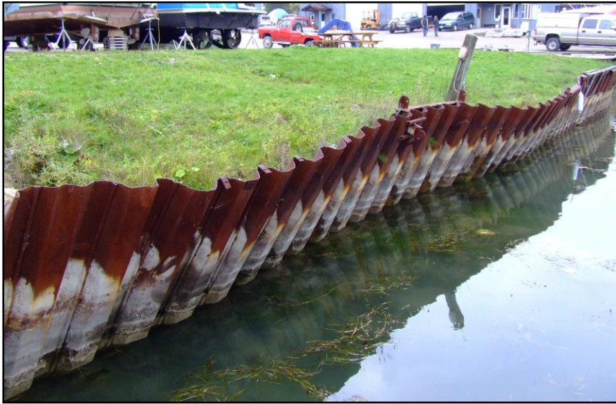
Figure 5.3.1: Subsiding sheet piling wall Photograph by Jordan Stewart
