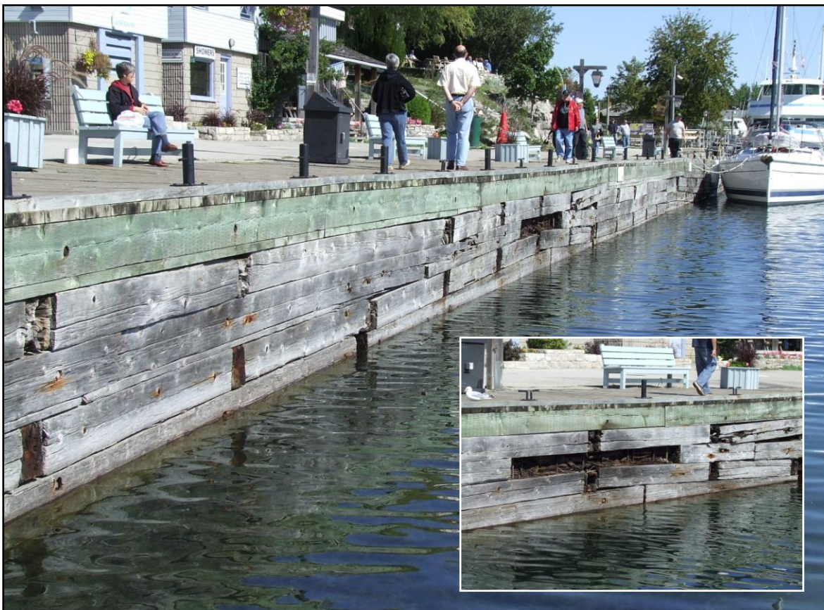
Figure 5.2.4: Illustrations of dry rot Photograph by Jordan Stewart
