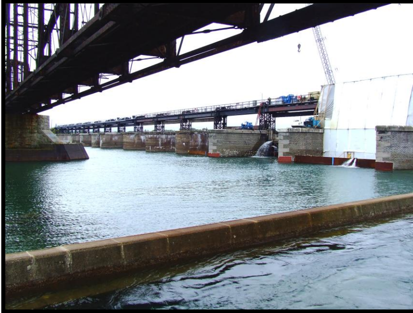
Figure 3.2.2: Outflow controls of Lake Superior Photograph taken by Jordan Stewart
