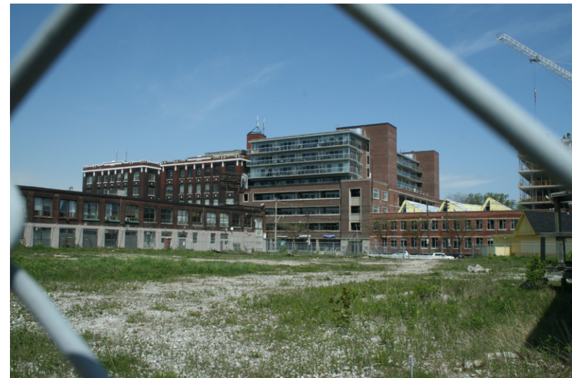
3.6. Industrial character of Carlaw across vacant lot of former Colgate-Palmolive factory.
