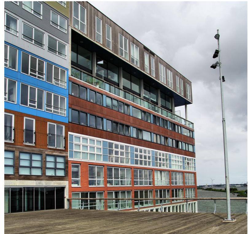
5.3. Silodam housing from main entrance deck.
