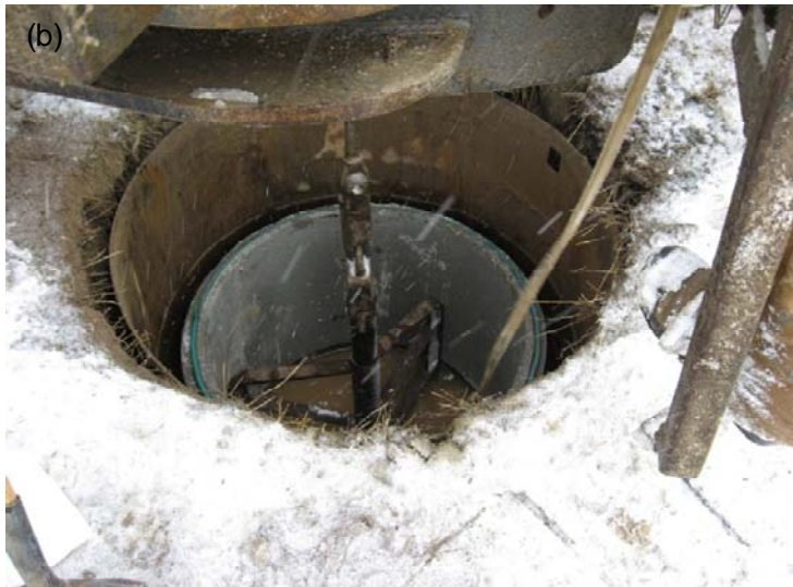
Figure 2.4. Large diameter test well installation photos showing (a) bucket auger rig, (b) hinged tile setter, (c) Poly – Lok lid with air filter, and (d) concrete cover and lid at CTH1.
