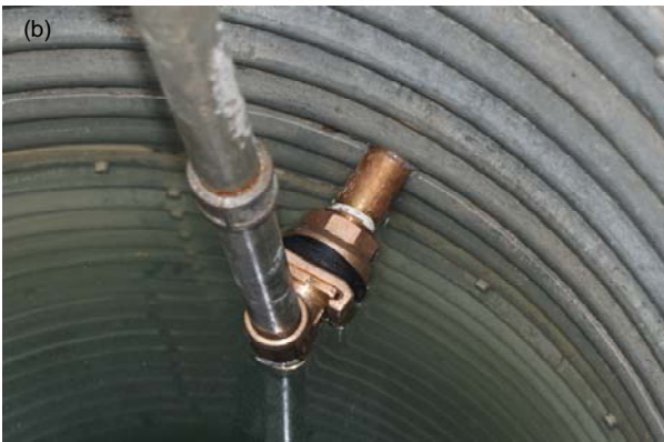
Figure 2.7. Pitless adaptor installation photos showing (a) placement of existing hydrated bentonite granules at ETH2, (b) pitless adaptor inside casing at ETH3, (c) pitless adaptor outside ETH3 covered with non-hydrated bentonite granules, and (d) pitless adaptor and non-hydrated bentonite granules covered with concrete to counterbalance the mass of the pump.
