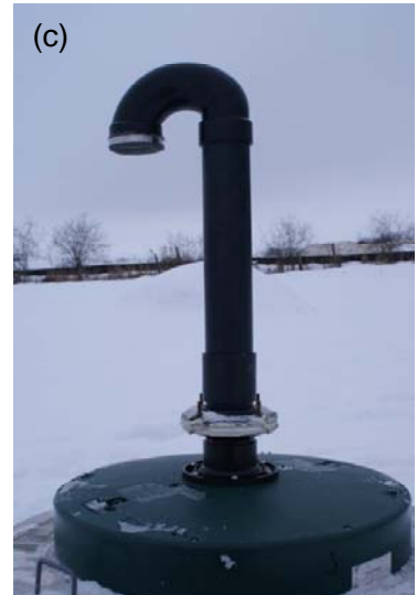
Figure 2.4. Large diameter test well installation photos showing (a) bucket auger rig, (b) hinged tile setter, (c) Poly – Lok lid with air filter, and (d) concrete cover and lid at CTH1.
