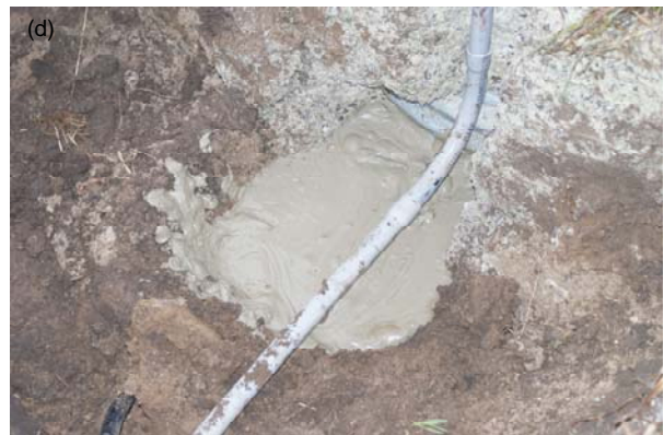
Figure 2.7. Pitless adaptor installation photos showing (a) placement of existing hydrated bentonite granules at ETH2, (b) pitless adaptor inside casing at ETH3, (c) pitless adaptor outside ETH3 covered with non-hydrated bentonite granules, and (d) pitless adaptor and non-hydrated bentonite granules covered with concrete to counterbalance the mass of the pump.
