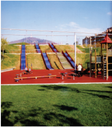
fig. 5.06 Playground built into the topography
