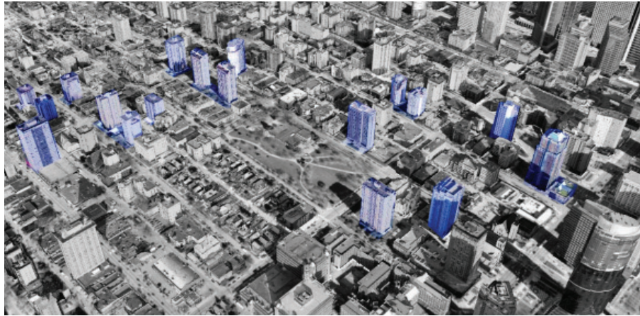
fig. 7.05 high rise buildings
