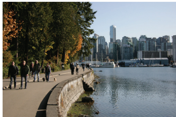
fig. 1.12 The seawall overlooking downtown
