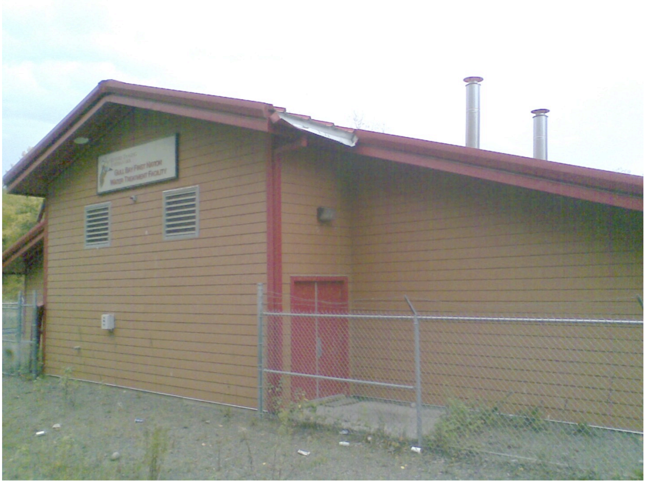
Figure 7: Gull Bay Water Treatment Plant (Inactive), in September of 2008
