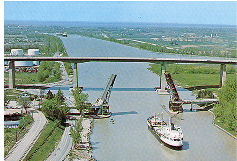
1.22 Garden City Skyway over Fourth Canal: c. 1983
