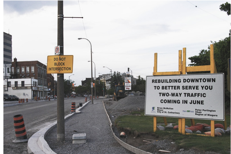
1.40 Road construction on St. Paul Street: c. 2009
