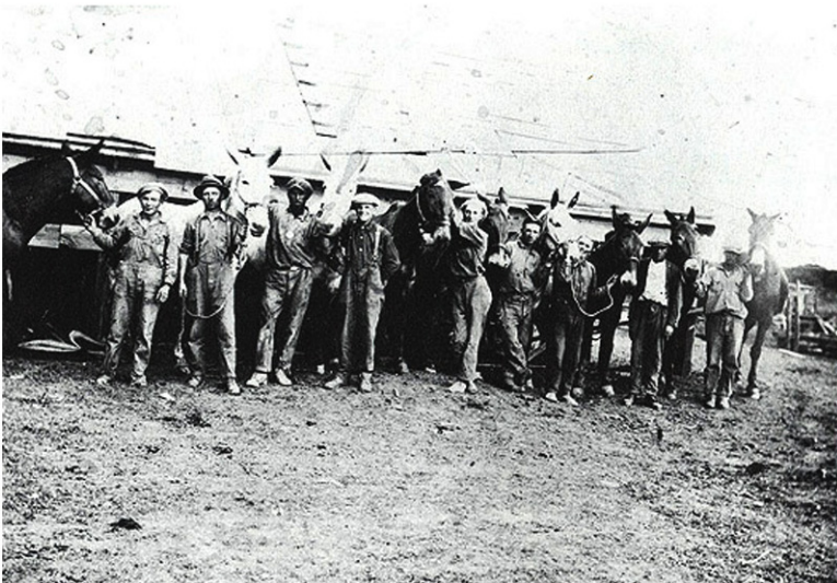
1.18 Fourth Canal construction crew: c. 1920
