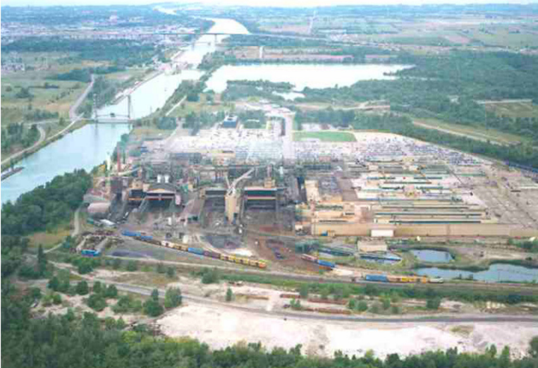
1.28 Aerial view of GM's Glendale Avenue Engine Plant: c. 1993
