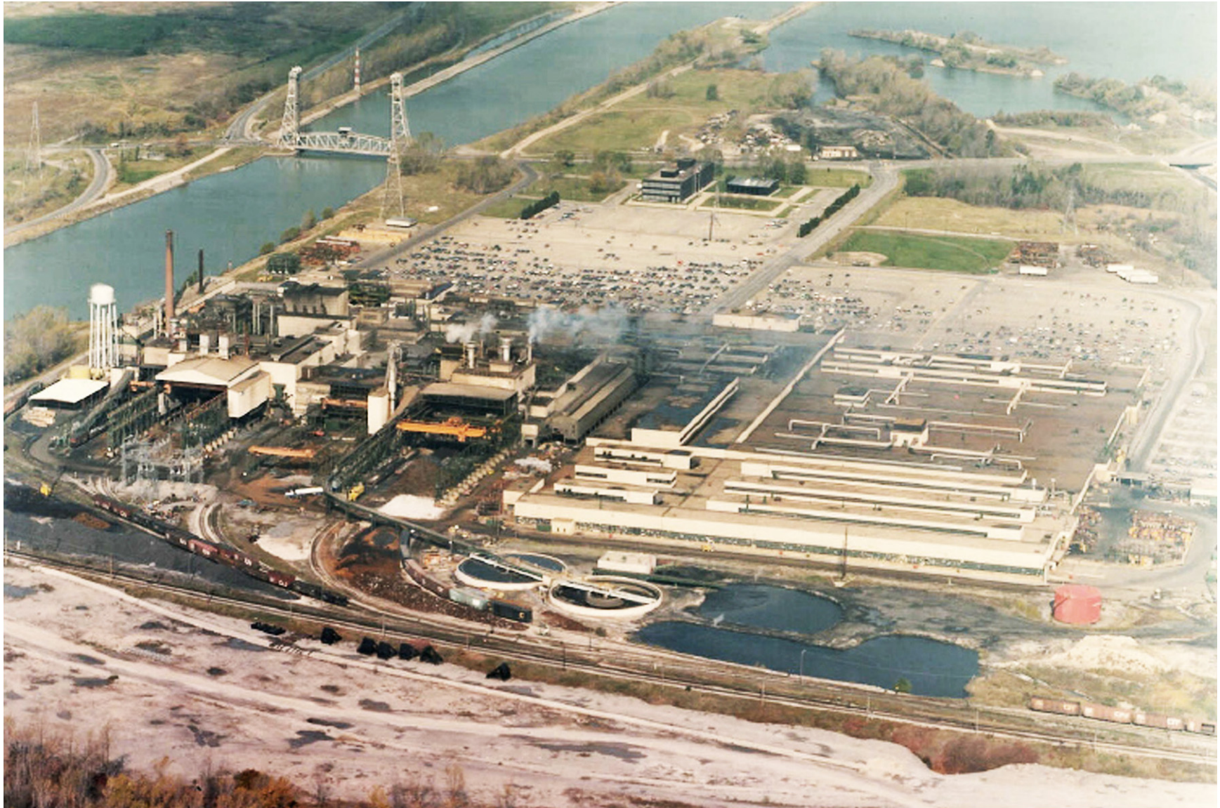
1.30 Aerial view of GM's Glendale Avenue Engine Plant: c. 1993
