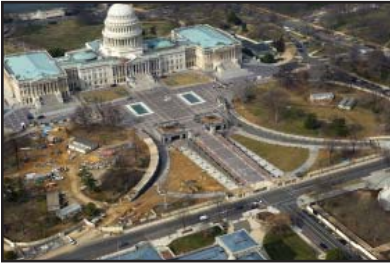
Fig 7.11 US Capital Visitor's Center UNDER CONSTRUCTION (2009) 124
