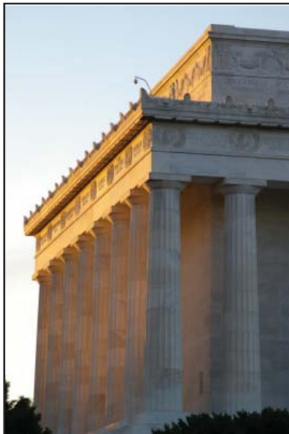
Fig 4.4 Doric columns of the Lincoln Memorial.
