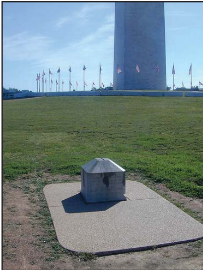
Fig 3.5 Photo of the Jefferson Pier in 2009. It was erected in 1804, and was built to mark the second prime meridian of the United States.
