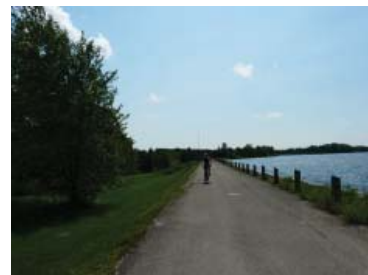
Figure 3.10 (above) Woolwich Reservoir Author's Photograph
