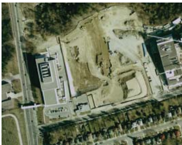
Figure 2.9 (above) Aerial Photograph of CNIB Google Earth
