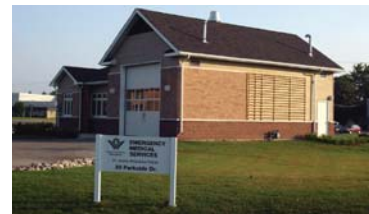
Figure 3.7 (above) St. Jacobs EMS Station Region of Waterloo Public Health 2009
