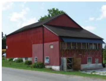
Figure 3.15 (far right) Garage and Gas Station Author's Photograph
