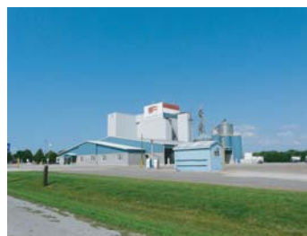
B The Floradale Feed Mill Ltd.
