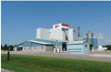
Figure 3.13 (above) Floradale Feed Mill Ltd. Author's Photograph
