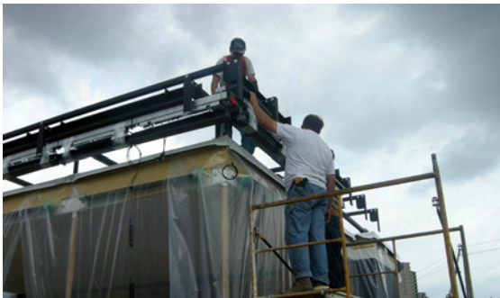
fig 2.12.1 installing the blinds
