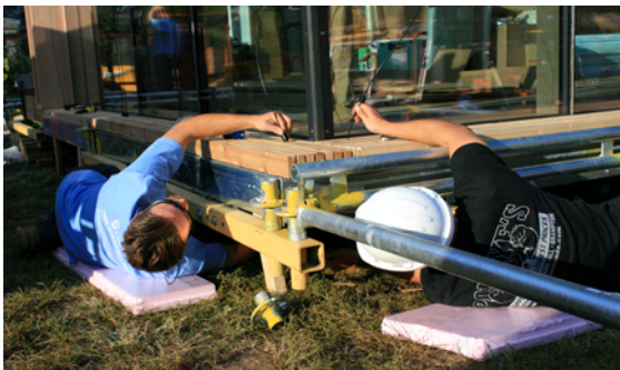
fig 2.12.4 installing the tension cables
