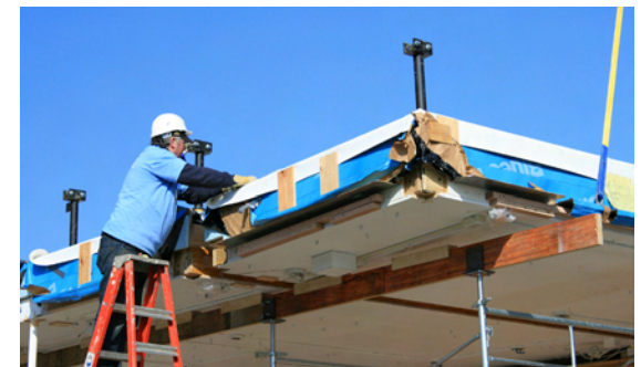
fig 2.4.6 temporary support beam used while placing roof panels
