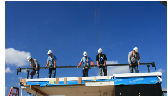
fig 2.5.6 placing the first roof racking frame
