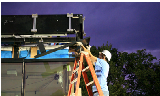
fig 2.9.1 installing the corner panel
