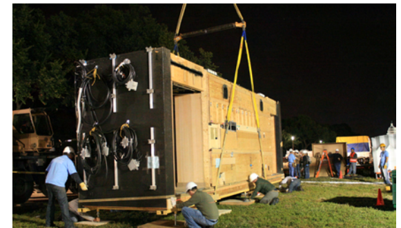
fig 2.2.4 placing the densepack
