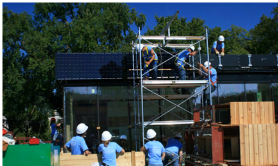
fig 2.13.4 installing the BIPV cladding panels
