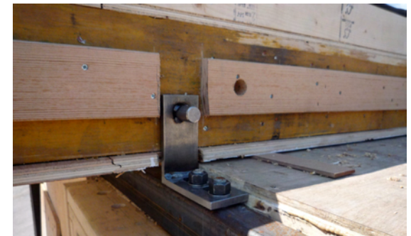
fig 2.4.14 angle bracket between roof panels
