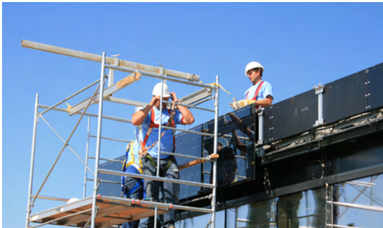
fig 2.13.1 hoist mounted atop scaffolding
