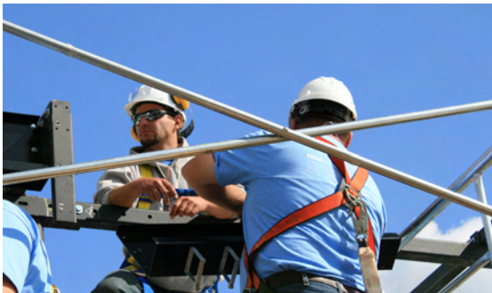
fig 2.10.1 installing the blind supports
