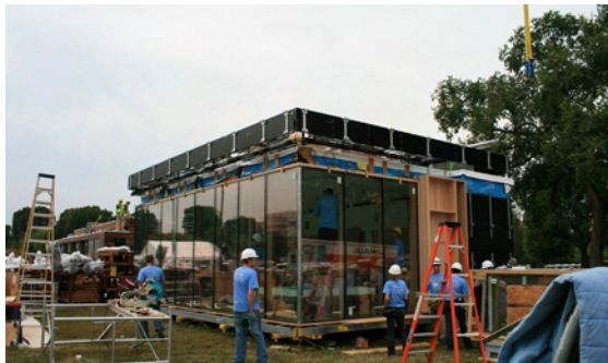
fig 2.8.1 The North House with glazing installed
