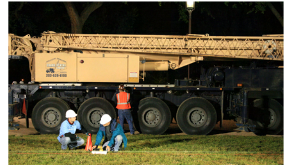
fig 2.1.4 setting out the string lines
