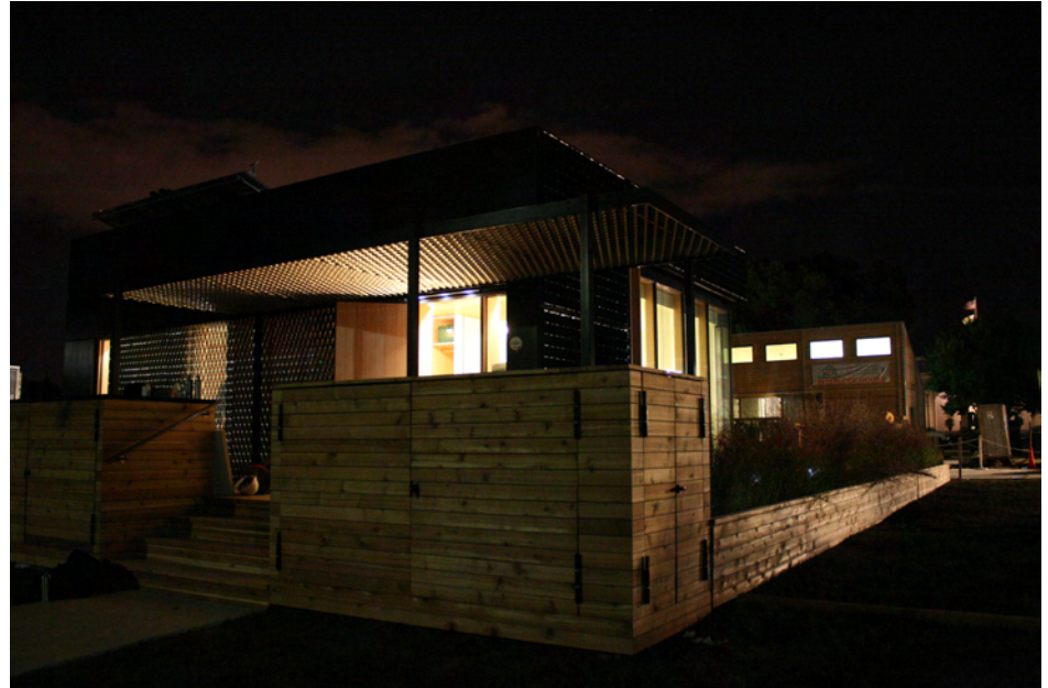
fig 3.5 The north main entry with canopy
