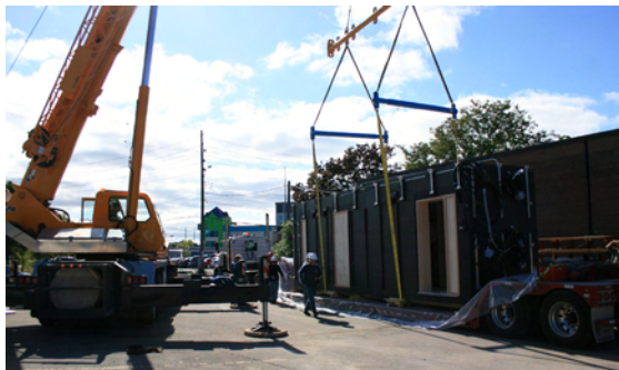
fig 2.2.1 crane rigging for the densepack
