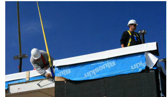
fig 2.4.13 tightening the threaded rods
