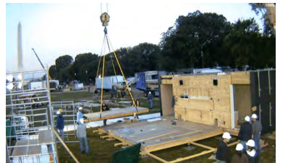
fig 2.3.7 placing the floor panels
