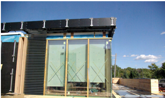
fig 2.11.1 cladding supports as installed
