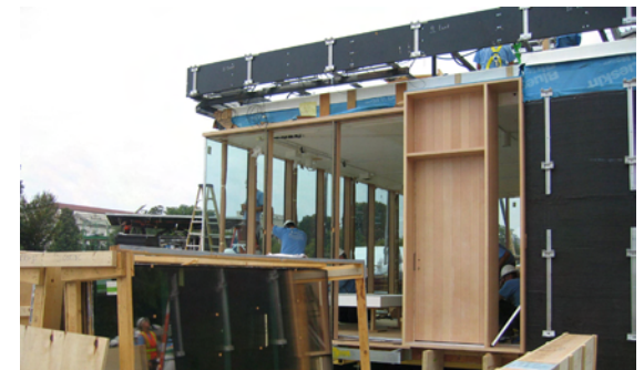
fig 2.6.10 The North House with mullions installed
