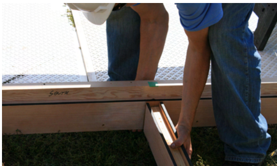
fig 2.6.1 connecting vertical and horizontal mullions
