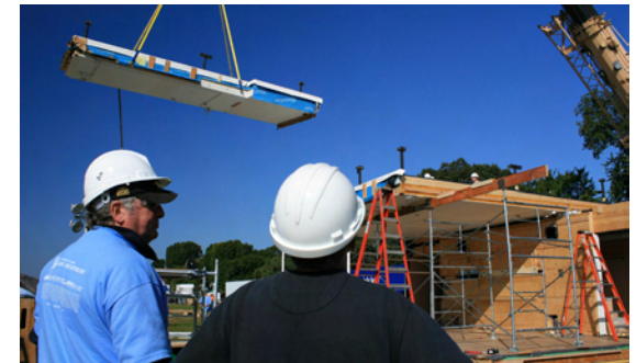
fig 2.4.5 placing the roof panels
