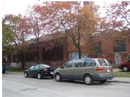
Fig. 3.13 90 Lisgar Street, Vacant industrial property.
