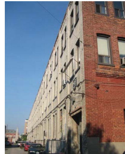
Fig. 3.2 48 Abell Street north lane way.
