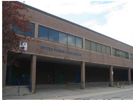
Fig. 3.7 6 Lisgar Street, United Foods Wholesale still in operation in 2005.
