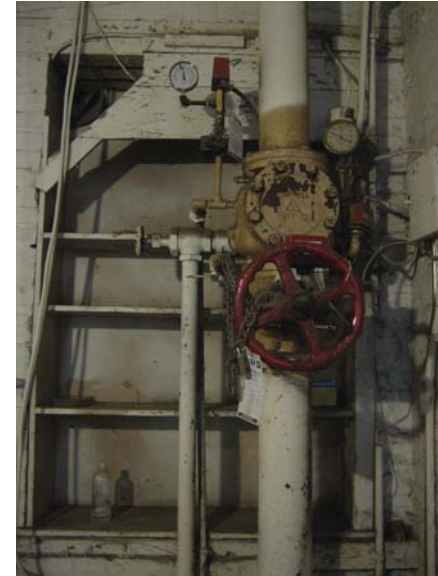
Fig. A.24 Above, Hissing pipes in the west wing corridor.
