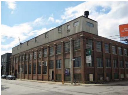
Fig. 3.12 40/44 Dovercourt Road. Site of Auto repair shops in 1970's.
