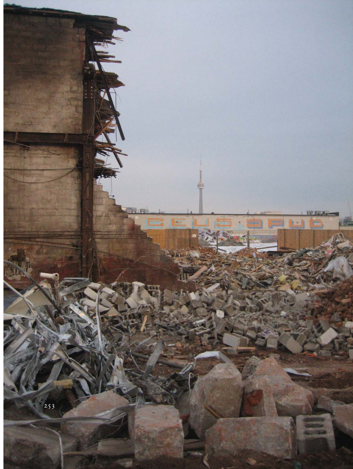
Fig. L.11 Right , CN Tower beyond 48 Abell construction waste.
